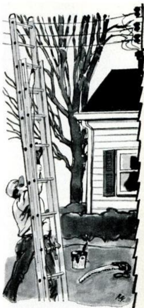
A power line and an aluminum ladder can make a deadly combination. Give yourself a safety margin; do not work any closer than 10 ft. from your power lines.
