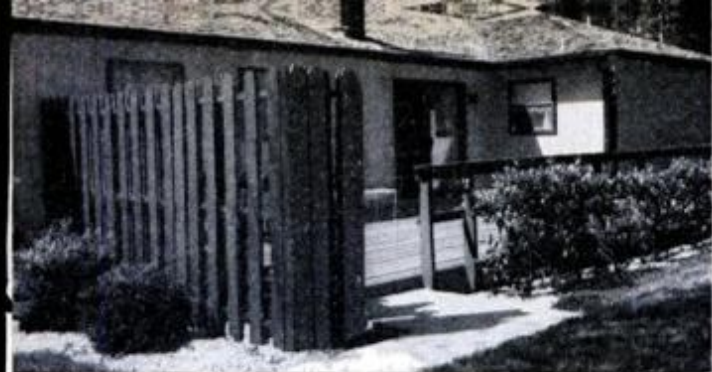
Tall picket variation has verticals nailed to both sides of three rails. Leave enough space between pickets and other types of vertical paneling to permit easy painting or staining.
