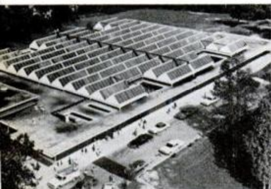
Already in operation, the nation's largest solar heating and cooling system is currently in use at the George A. Towns Elementary School in Atlanta, Ga. Over 50 A-shaped rooftop solar collectors supply more than 60 percent of the school's heating and cooling needs. Reflectors on back slope of each unit allow collectors to absorb energy from both direct and reflected sunlight for maximum efficiency.
