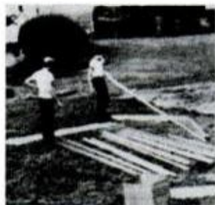
1 To erect this Janco unit, first sort the parts.
