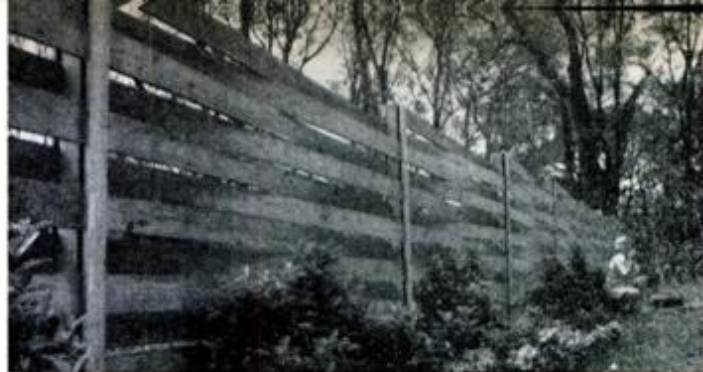
Paneled and louvered fences on pitched grades are easier to construct in a stepped sequence than canted to fit a hillside. Picket and post-and-rail fences are more suited to the contours.
