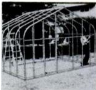
5 Install the gable ends to the freestanding unit.
