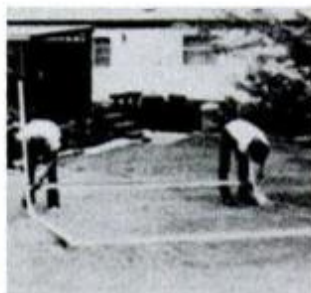
2 Assemble the frame from base, working upward.
