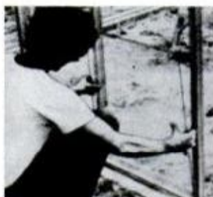
9 Repeat steps 7 and 8 for the rest of the glazing.
