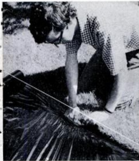
After you've rolled out black plastic, tuck its edges under the sod in small trenches you've dug. Sod anchors the plastic.
