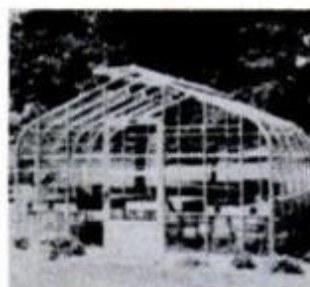
10 Completed unit with benches ready to paint.
