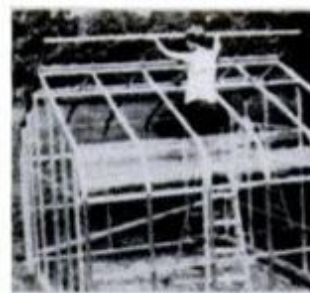
6 Next, add the roof sash to the greenhouse.
