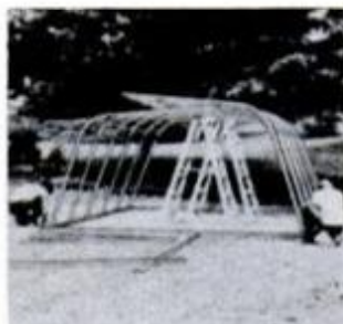
3 Place the frame on a permanent foundation.
