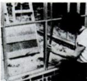
8 Lock the glass in place with bar cap and screws.
