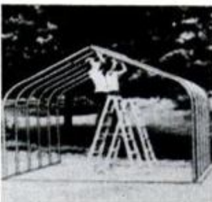
4 Attach the ridge and sill sections together.
