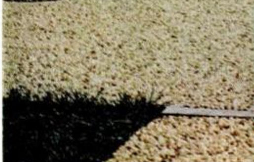
Stones bonded together with epoxy make an attractive, easy-care, nonskid surface. Designed by Astro-Stone, Brooklyn, N.Y., the covering is professionally installed.
