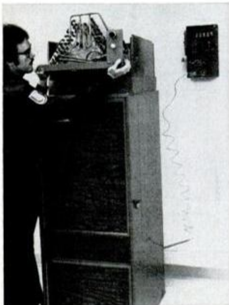
Indoor coil of York MaxiMizer add-on heat pump fits onto a fossil-fuel, forced-air furnace like an airconditioning coil.
