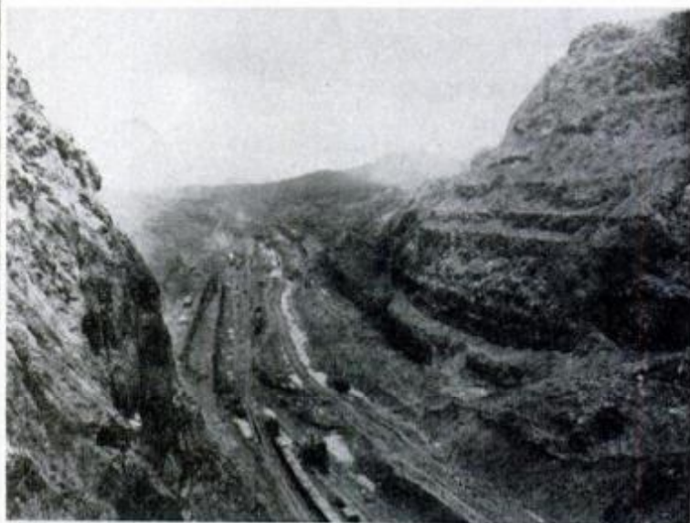
Instability of Isthmus soil is a problem facing engineers even today, as it did during construction of the present canal. In the continental divide, mountainsides tumbled into excavation (above). Among other precautions, extensive drainage systems protect some sections (top, right). The spectacular Gaillard Cut (formerly called Culebra Cut) through continental divide claimed many thousands of lives and caused endless grief as material from steep sidewalls kept sliding into deep channel.
