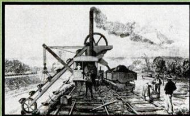
Canal project saw development of earth-moving giants . . .
