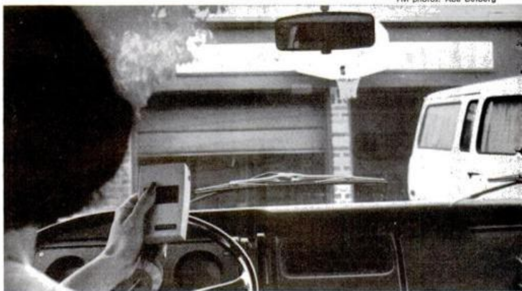
One touch on transmitter button raises garage door; another closes it again.
