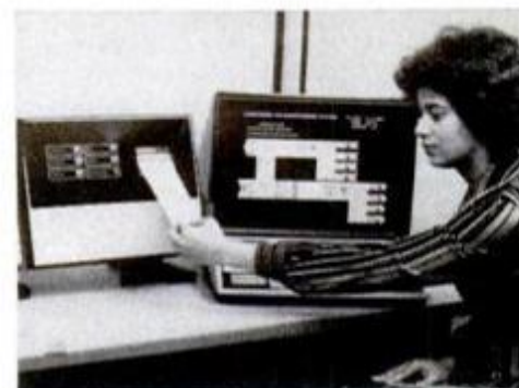
Desktop control center for Honeywell's energy management (and/or fire-security) system programs power-use needs.
