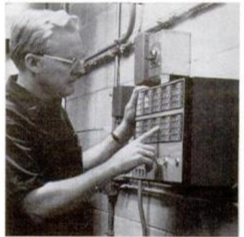
Unit at right performs the switching operation in private homes in Cedar Grove and Belgium, Wis., involved in a load-shedding operation designed by the local utility company to level peak loads.
