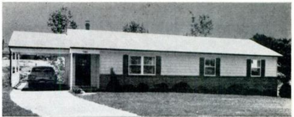
Energy-efficient house is a normal-looking ranch. At its front—north side of house—(above) only clue to its nature is reduced window area. At its rear—south side of house—(left) there's extra window space protected from summer sun by broad-leaf trees and 2-foot roof overhang.
