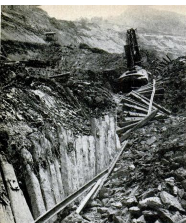
Instability of Isthmus soil is a problem facing engineers even today, as it did during construction of the present canal. In the continental divide, mountainsides tumbled into excavation (above). Among other precautions, extensive drainage systems protect some sections (top, right). The spectacular Gaillard Cut (formerly called Culebra Cut) through continental divide claimed many thousands of lives and caused endless grief as material from steep sidewalls kept sliding into deep channel.
