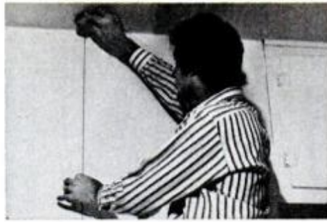
2 Measure for first strip at a door or window; the edge overlaps \frac{1}{2} in. Snap a chalkline where the other edge falls.
