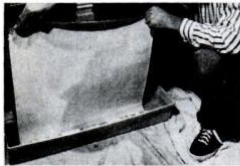
4 Hold the bottom edge; roll the strip, paste side out, in the filled water tray. Weight it down with a table knife inside.
