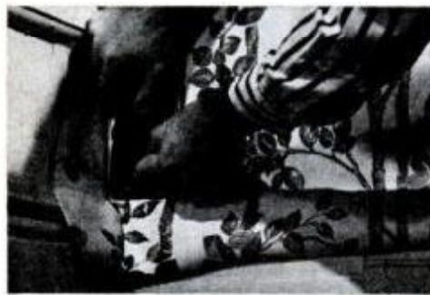
7 Unfold and align bottom. Smooth with a brush. Use putty and razor knives to trim the paper at ceiling and baseboard.
