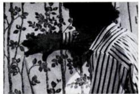
9 Dip and hang the next strip. Match the pattern carefully while you work. Butt the edges and sponge off the paste.
