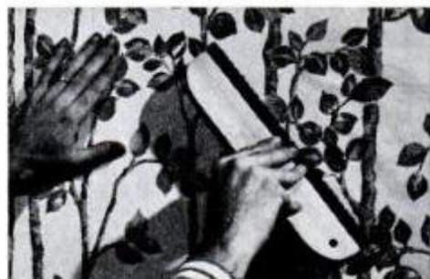
11 Wallpaper brush smooths large air bubbles. Work from center outward. Small bubbles will disappear with drying.
