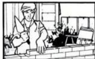
Lay brick with speed and precision!
