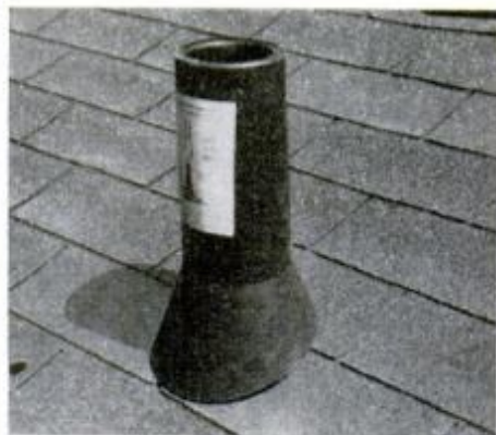
Base can be trimmed to suit roof's pitch.
