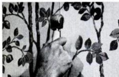
10 A seam roller is used to secure the edges. However, on both flock and foil coverings tap seams with a sponge.
