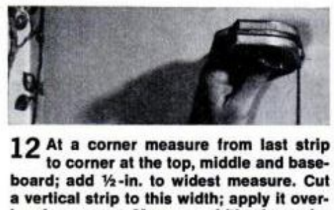
12 At a corner measure from last strip to corner at the top, middle and baseboard; add \frac{1}{2} -in. to widest measure. Cut a vertical strip to this width; apply it overlapping corner. Measure width of remaining strip, add \frac{1}{2} -in. and drop plumb this distance from corner to guide hanging first strip on remaining corner wall.
