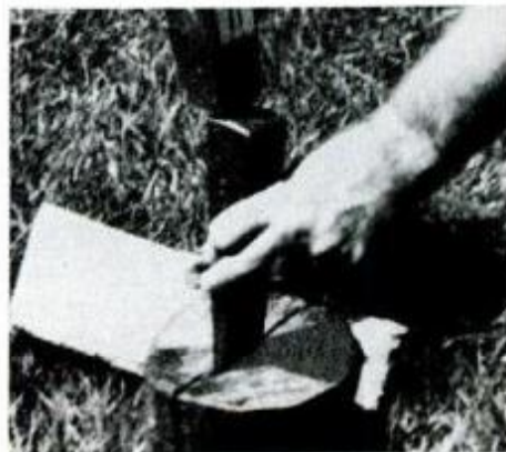
Wedge is driven with hammer end of head.
