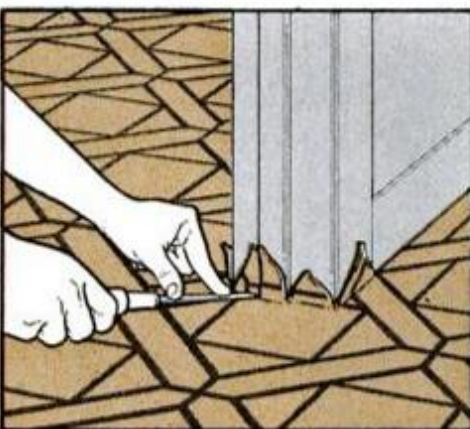
Holding screwdriver flat, press vinyl into the angle of the floor and doorway trim.
