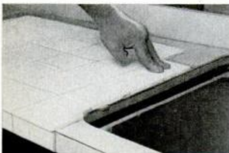
7 Install additional tile, cut to meet edge wherever it's necessary.
