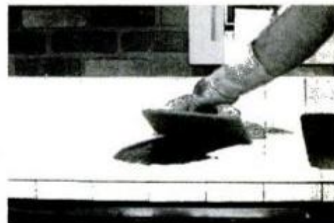
15 Spread grout liberally over all tiled surfaces with a rubber-faced trowel.
