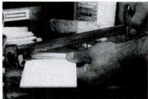
10 Scored tile breaks cleanly under pressure on both sides of cutting line.
