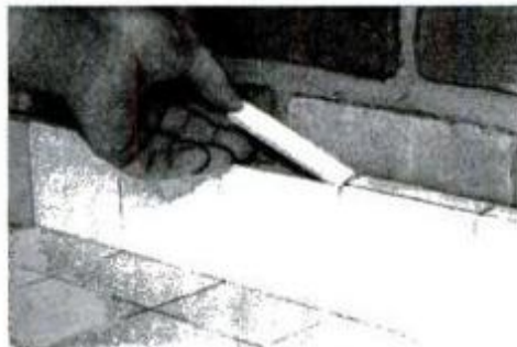
11 Strips butt against the backsplash tiles to form a square corner.
