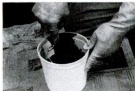
14 Then mix the grout with water according to manufacturer's directions.
