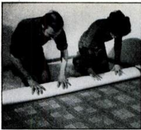
To "relax" the flooring, roll it, backing side out. Roll it once from each end.
