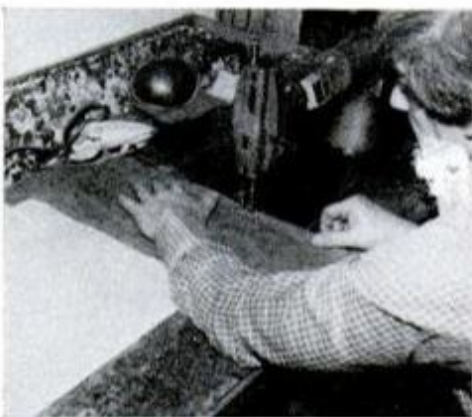
13 The pull strips help to position the fabric to produce a tight fit.
