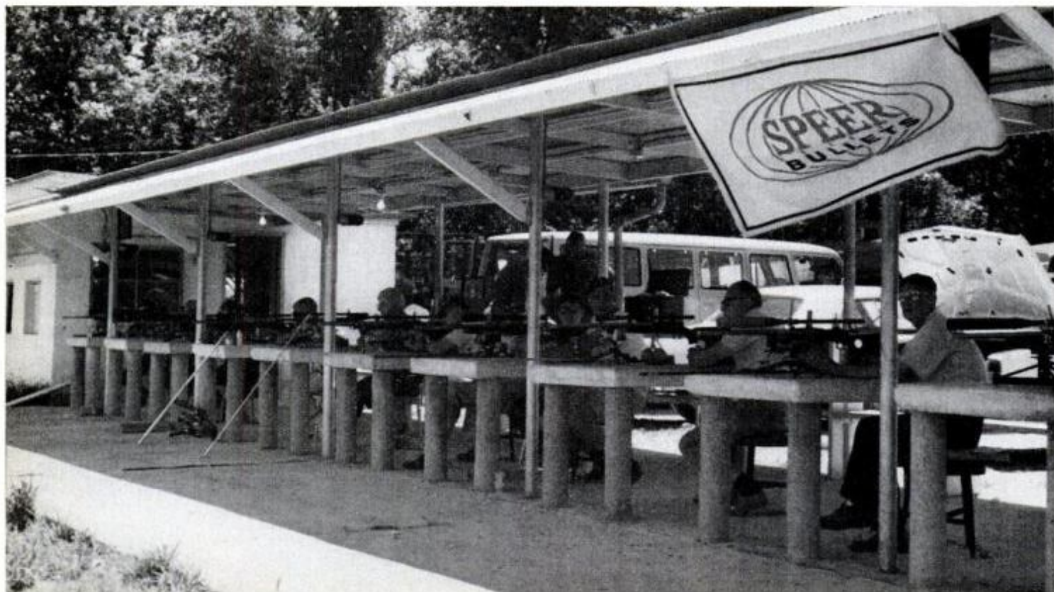
For bench-rest competition, massive reinforced-concrete benches of special design provide solid support for weighty rifles.
