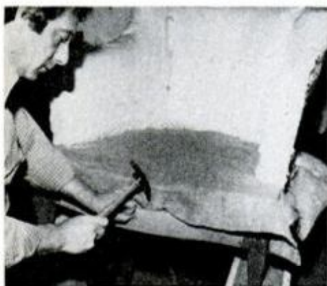
8 Tack burlap over the seat springs, then sew it to the top of the seat.
