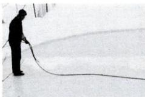
On a large rink, it's best to water back and forth in sections approximately 6 ft. wide across the width of the pool.
