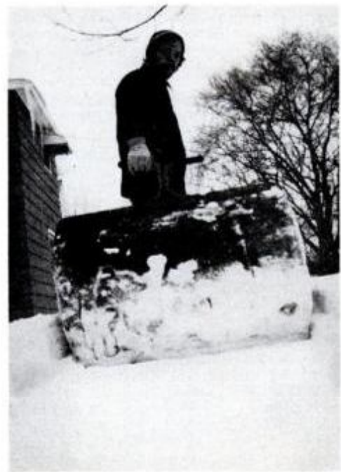
A base of more than 4 in. of snow will have to be packed down. It's more easily done with a lawn roller than with feet.
