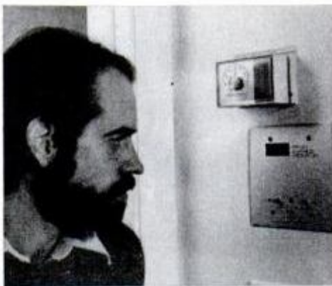
Entire device, except for transformers that act as sensors, mounts flush in wall, usually near thermostat, to make a total energy control center.
