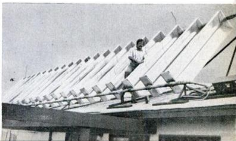
John Kusianovich of Albuquerque, N.M., chose to use an array of concentrating collectors that track the sun for his system.
