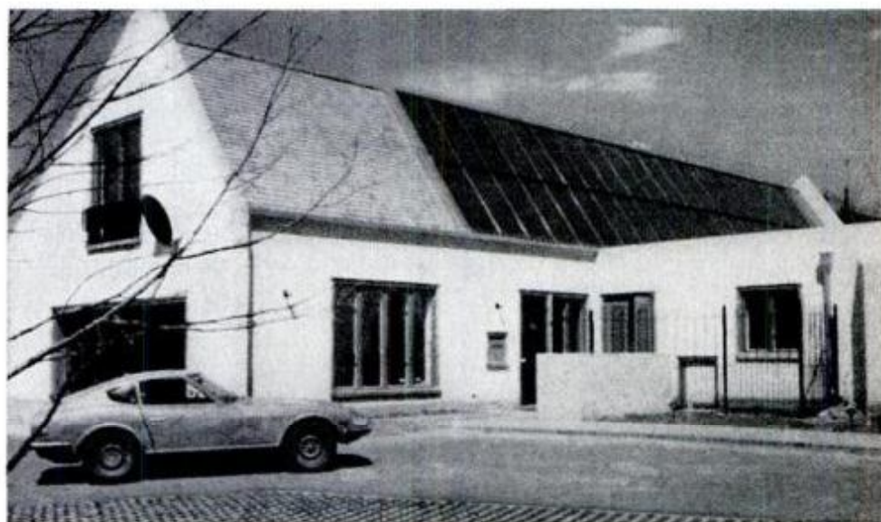
Architect James Sudler's 5800-square-foot Denver home has an air system that provides approximately 70 percent of the space heat and domestic hot water needed. The total bill for this large-scale system came to approximately $20,000.
