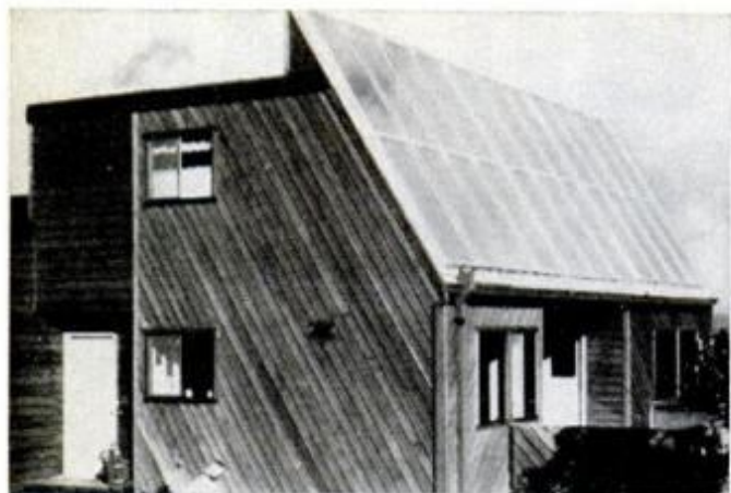
Solar system in the home owned by the Douglas Boleyns of Gladstone, Ore., was installed as a demonstration product by Portland General Electric at cost of $30,000—much of this was accounted for by monitoring equipment and conservative design.
