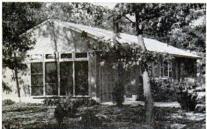
Charles Marsh of Pomona, N.J., spent $1500 to add air-cooled collectors to a vertical wall of his home. The system takes care of one-third to two-thirds of his space-heating needs.
