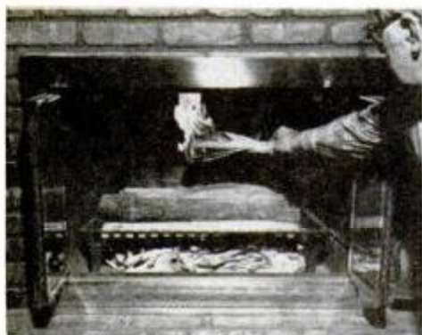
Light paper under open damper to create updraft; then light kindling under grate.
