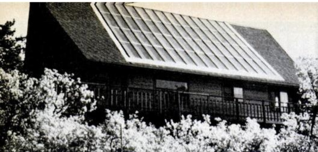
Heightened awareness of the country's present and future energy problems got Bruce Robinson into solar heating—he made his decision while energy chairman of the Sierra Club. The air-type system in his Morrison, Colo., home cost $7000.
