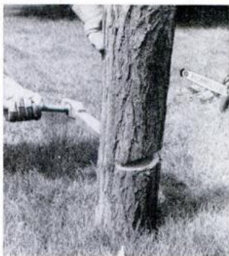
Cut the back cut 2 in. short of the notch; then push or drive wedge in the backcut.
