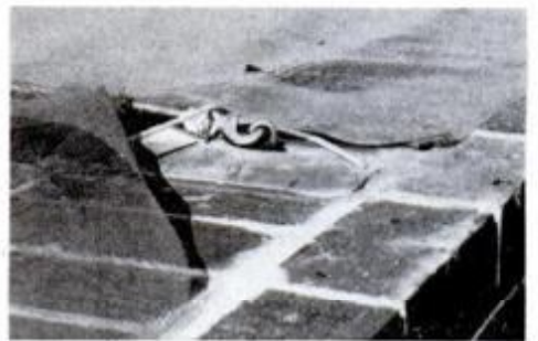
Fiberglass-screen cover admits plenty of sunlight to pool and deck. Below, snap hook and eye anchor support line to wall.
