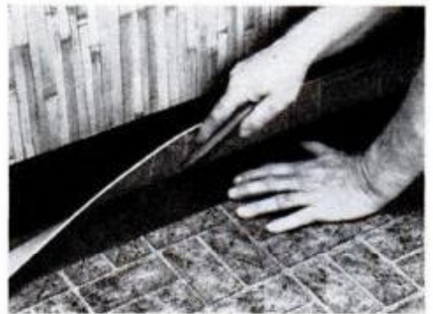
Second, trim the material along the room edges with a knife and straightedge guide.
