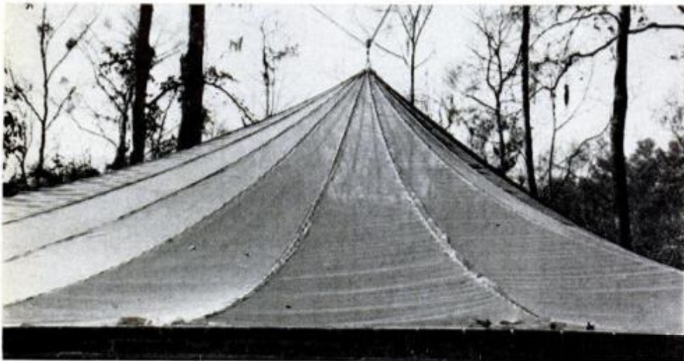
Fiberglass-screen cover admits plenty of sunlight to pool and deck. Below, snap hook and eye anchor support line to wall.
