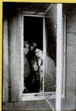
6. WINDOW LOUVERS Adjustable mini-louvers between double-glass panes block heat of the summer sun.
