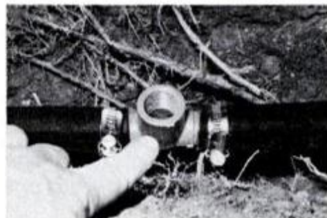
A tee fitting attaches to the flexible pipe with hose clamps. Next the riser pipe and the sprinkler head are installed.
