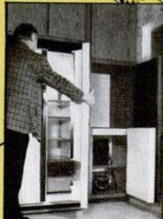
5. REFRIG. HEAT BOX Refrigerator heat goes out in summer, inside in winter.
