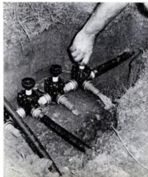
A tee fitting attaches to the flexible pipe with hose clamps. Next the riser pipe and the sprinkler head are installed.
