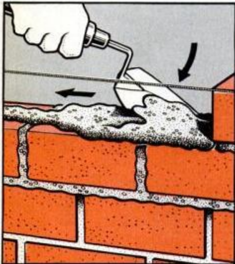
First, with a trowel , spread the mortar evenly, adding slightly more than needed. Use mason's line for accuracy.
