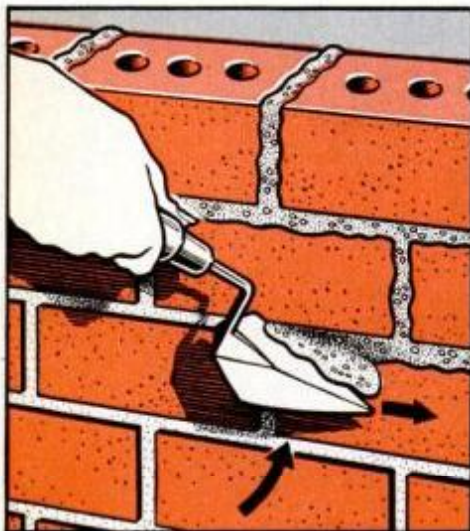
Third, remove mortar squeeze-out with your trowel and return it to the mortar tub so you can use it again.
