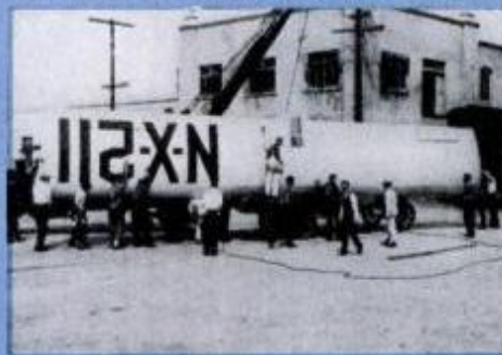
Oversize wing for the Spirit was built on top floor of Ryan factory (above). To get it out, workers slid it out to the roof of a freight car on the siding, then hoisted it to a flat-bed truck. At right, craftsmen assemble ribs 11 inches apart to insure airfoil contour integrity.
