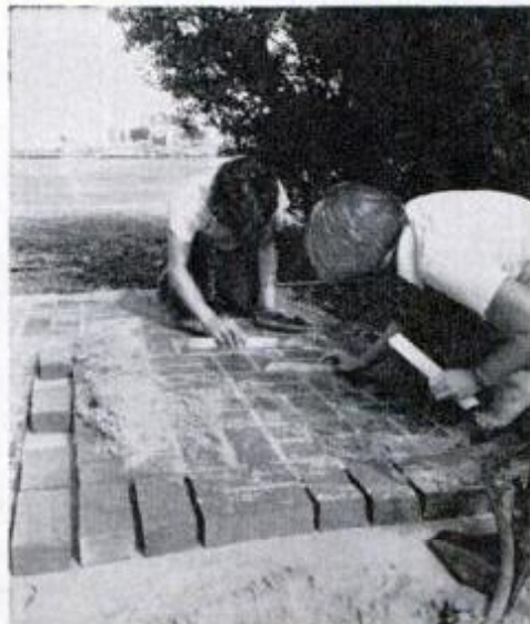
Lay the bricks close together and sweep sand between the joints. Then wet the sand down to compact it.
