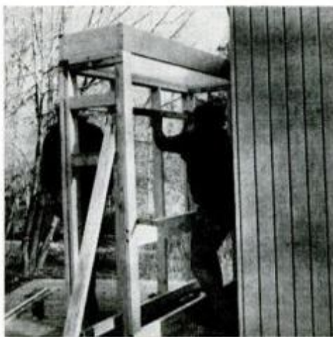
Lighten the weight of the shed (as well as the load on the casters) by the use of 2x2 shelf nailers across the back.
