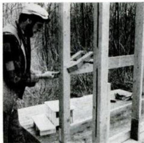
Use a clamp to hold the 2x6 flush when turning the lags. Add 2x4 nailers above for as many plywood shelves as you want.
