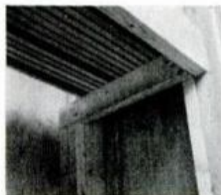
Complete the door by running 2x4 nailers from the back wall studs to the front 2x6 to support 1x2 redwood slats (on edge
