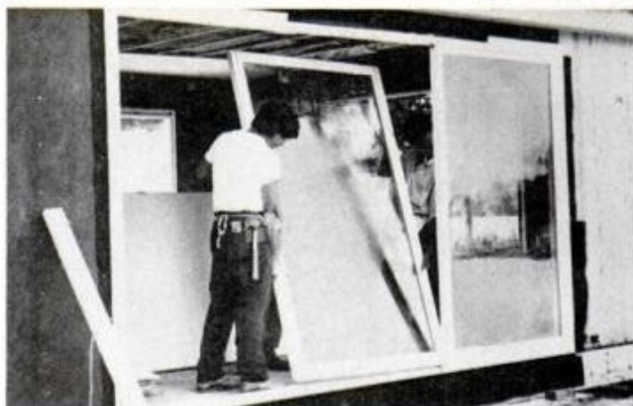
Adjustable rollers on the operating door ride on a rib in the sill. A vinyl thermal barrier runs the length of the sill.
