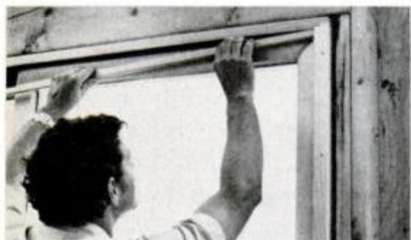
Head stop screwed to head jamb completes track for the doors. Rollers can be adjusted for height.
