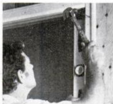
Nail casing through sheathing into studs with 10d casing nails.
