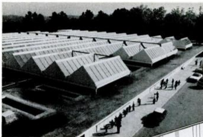
Twelve rows of collectors totaling 10,000 sq. ft. constitute one of the world's largest liquid-system installations atop elementary school in Atlanta, Ga. The 576 PPG flat-plate units handle more than 60 percent of the heating and cooling load.
