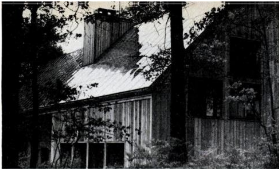
Still think solar collectors have to be ugly? This beautiful conference center on New York State University campus at Albany uses 2300 sq. ft. of flat-plate collectors and a 25-ton heat pump. Two 8000-gallon tanks are used for storage.
