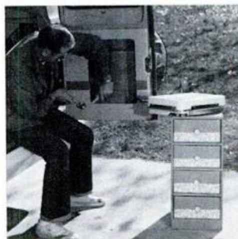
Balancing act allows hookup of lines and securing heater with sheet-metal screws.
