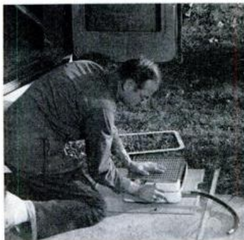
Shape of heater is traced on pattern for marking and sabre-cutting the van door.
