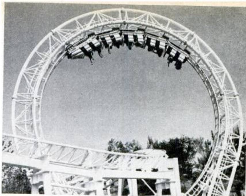
Vertical loop, spiraling turns, steep drops and a long tunnel section are features of this 3657-foot, 50-mph ride at Magic Mountain park in Valencia, Calif.
