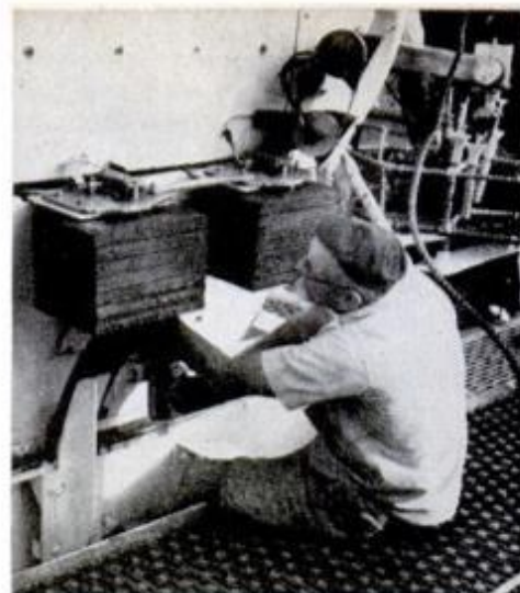
Back from dive, Alvin is carefully guided into stern well of mother ship Lulu for retrieval in a cradle (left). Above, a technician checks diving weights—stacks of steel plates each weighing 230 pounds—that can be released to control buoyancy.
