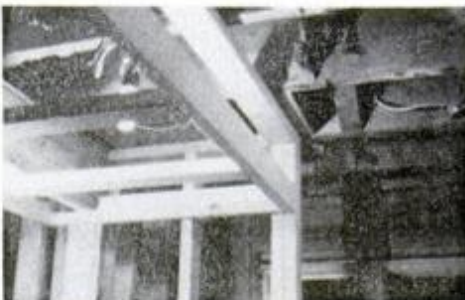
Framing in. A new dropped ceiling joins the partition separating the tub and the toilet. The one-piece unit fits inside.
