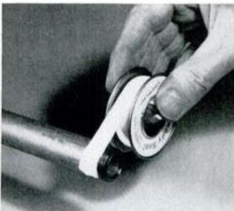
The Teflon tape is wrapped around male pipe threads to lubricate and seal.
