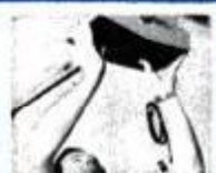
2. Attach power unit to ceiling.
