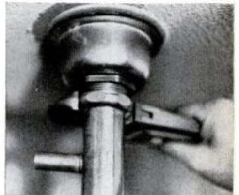
12. Drainage. This 1 1/2-in. drain line has a presoldered tee for clamping on the end of the dishwasher drain hose.
