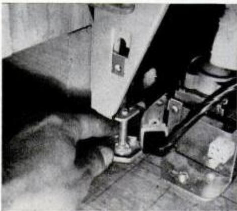
13. Leveling. Slide the unit into the opening over the control box. Unload (lift up) to adjust the leg height.
