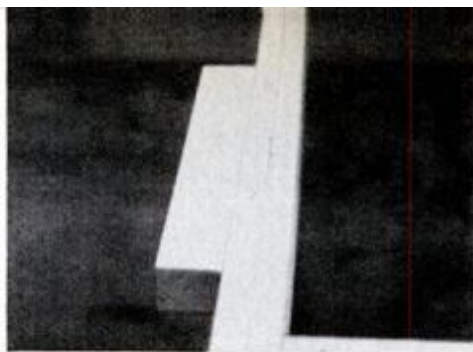
2. Extra support. A 2x2 block added to the cross brace makes the counter stronger. Pre-drill it for 2-in. screws.
