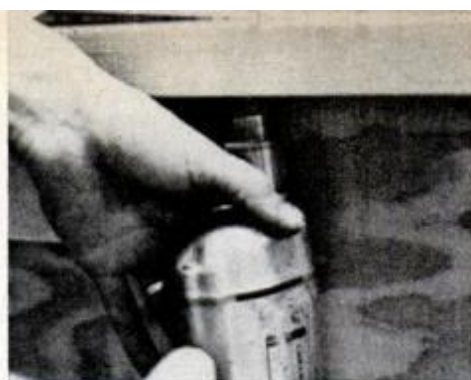
1. New counter rails. We screwed new 2x2 rails along the back wall (and predrilled them) to support the counter.
