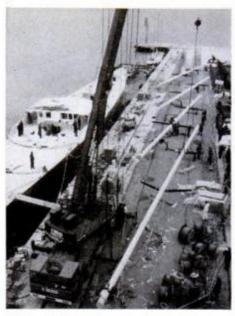
Masts of 98 feet fore and aft, 105 feet for two amidships, lie ready for stepping. They are balanced by depleted-uranium keel.
