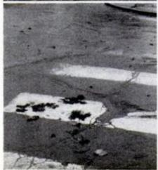
Keep your eye on the road surface: At far left, the slipperiest part of the uphill stretch is in the middle where there's an oil slick from vehicles and trucks laboring to the top. Top left is an asphalt surface: it's slippery, but tires get some bite on the high spots. Center left is classic hazard of wet leaves on turn. Bottom left is a combination of slippery surfaces: leaves on shiny. smooth crosswalk markings, and loose pieces of broken pavement that further increase the danger.
