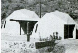
Geodesic domes (above) are simple, efficient, easy to build, economical. Stock 2x4s fit into ring connectors that automatically align 2x4s at the proper angle. Sizes vary from a small 18-ft. model up to giant 49-ft. dome. For a free catalog, write Dyna Dome. 22226 North 23 Ave., Phoenix, Ariz. 85027.
