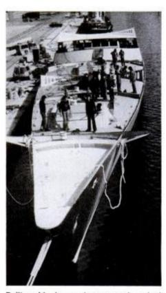
Built upside down, schooner was launched inverted with deck sealed. Skin divers then opened hatches in deck while cable-pull on keel righted hull, shown below.
