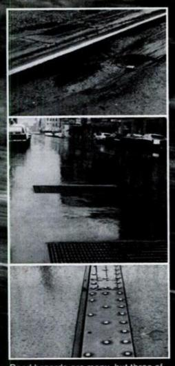
Road hazards are many, but three of the most dangerous are shown above. Railroad tracks should be crossed at right angles, and watch for washouts alongside tracks. Gratings come in all shapes and sizes and are slippery; so are expansion joints.
