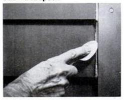
After you run a bead of caulking along the casing of a door or window, dip a plastic spoon in turpentine and run it along the bead. You'll wind up with a crack that's fully packed and a neatly tooled fillet.
