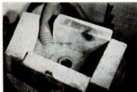
Add sand, level with elbow opening, then set four firebrick on edge around opening.
