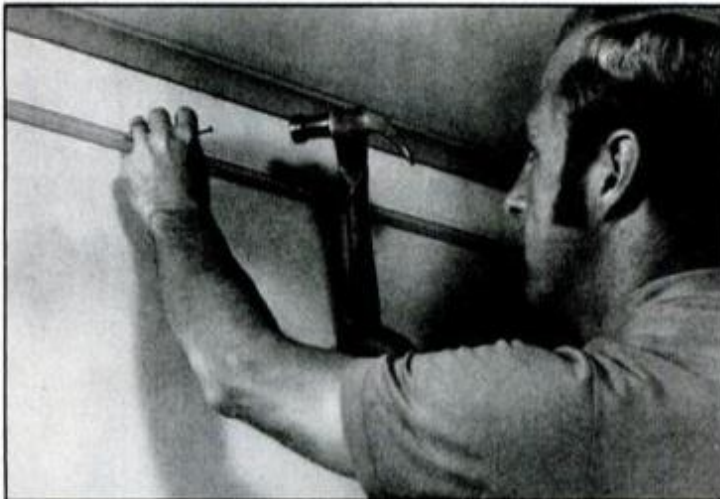
1. When you install suspended ceiling, chalk new ceiling height around perimeter of room. Nail metal molding to studs along line.
