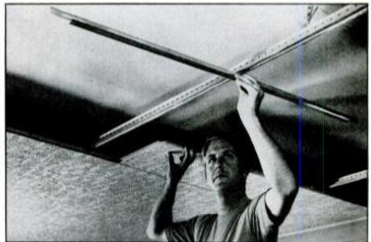
4. First 1x4-ft. tile (or four 12x12-in. tiles) rests on wall molding. Cross tee snaps on runner, slides into slotted tile edge.
