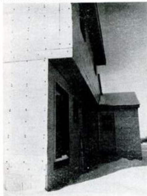
Dow Chemical, 1880 Mackenzie Drive, Columbus, Ohio 43220, has developed a code-approved, one-inch-thick, Styrofoam sheathing. It's applied to all exterior surfaces, including foundation walls below grade. It does such a good insulating job on its own that conventional 3½-inch batts in the wall become more efficient. You can carry about twelve 4x8 sheets under your arm quite easily.
