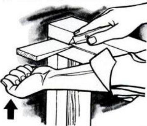
Trim off the excess so that the edge will remain flush for Sheetrock or siding.
