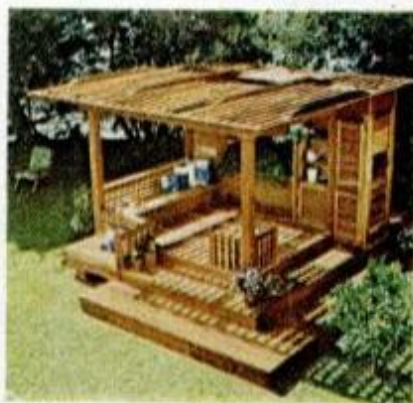
The trellis roof is made up of 2x2s in frames. Use them for filtered light or use plywood for shade.
