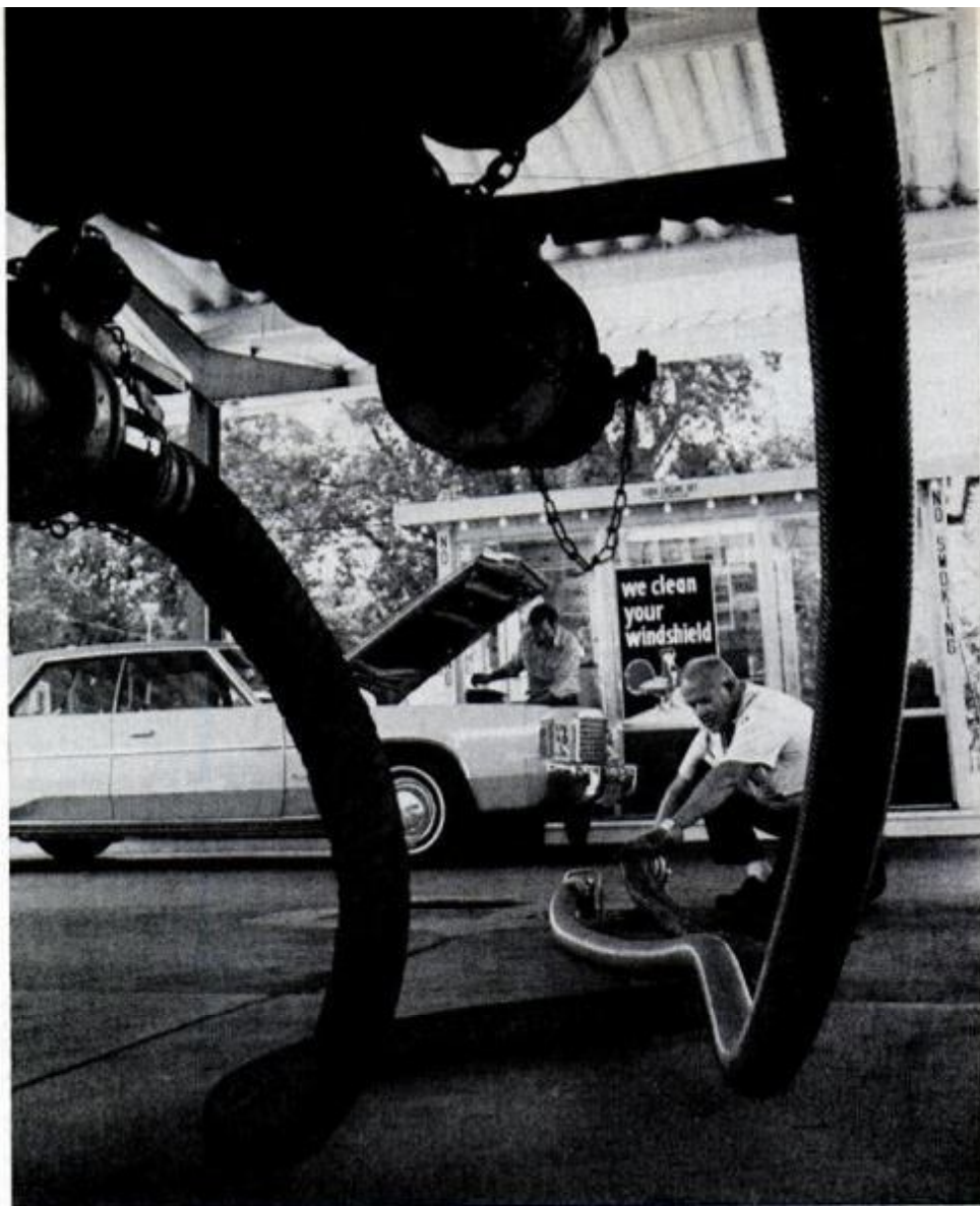
LOADING TANK TRUCK
