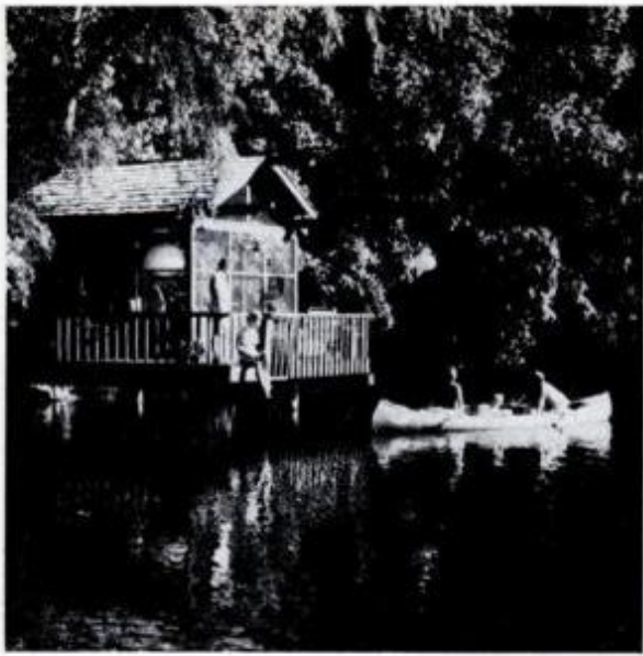
Screen house: Pilings are used for support in this unique setting. The design beats mosquitoes in back yards, too.
