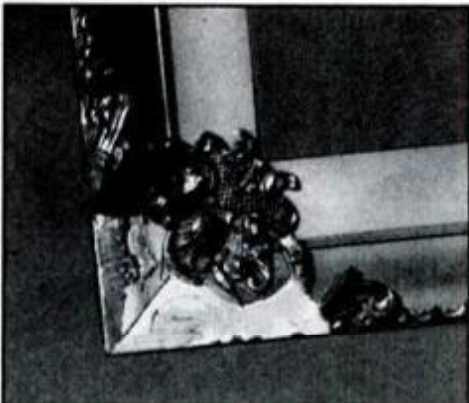
8. When this much of embossed overlay is missing, the overlay must be replaced with a new casting. It's beyond repair.
