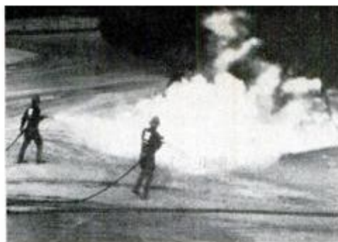
Double-teaming a fire —a standard industrial and military practice—two instructors advance together (above), aiming hoses at edge of flame and sweeping side to side so streams overlap slightly. Fire (below) is out in seconds; only smoke remains.
