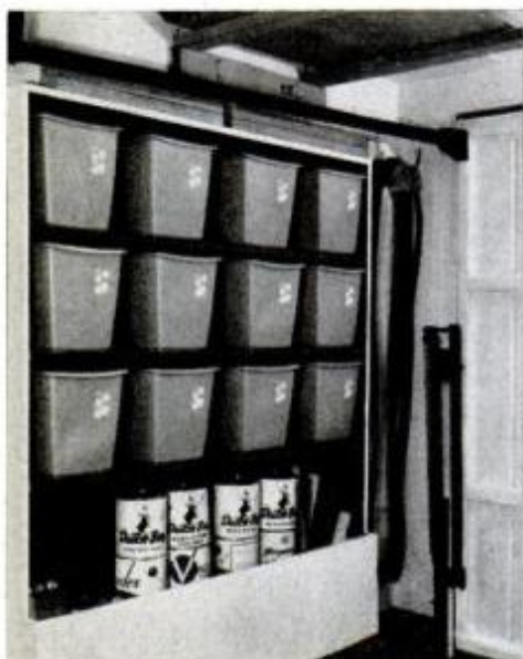
Shelves are recessed into the wall studs for neat and efficient storage.
