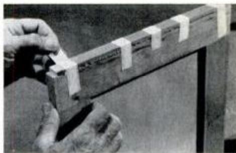
Corner notches are formed by gluing short 1/4-in.-thick strips to the front edges.
