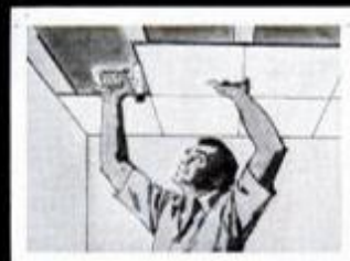
Put up ceiling tile.
