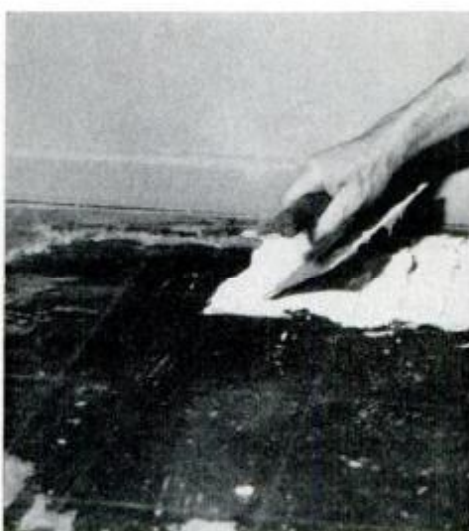
Next, low spots and cracks are filled with GAF's Flor-Fix, which dries quickly.
