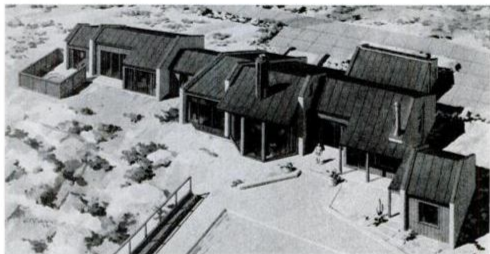
Decade 80 House , experimental solar home of Copper Development Corp., features sprawling, irregular layout to break up appearance of its many copper-coil roof collectors. System also heats attached swimming pool.
