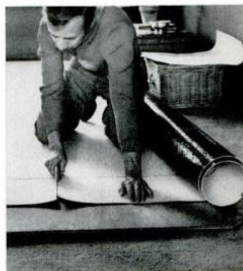
Using a sharp utility knife, sheet vinyl is cut slightly larger than room size.
