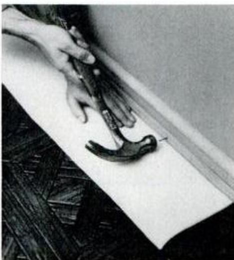
Scrap of vinyl maintains expansion gap above flooring as shoe mold is replaced.
