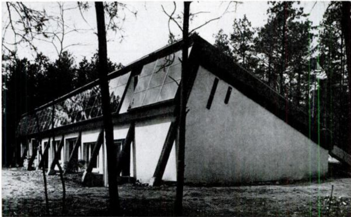
Stylish Homan house in New Jersey proves solar homes don't have to look like greenhouses. Array of collector panels angled across front has handsome look of large picture windows. Typical panel, devised by solar pioneer Harry Thomason, is shown at left, below. Water flows down corrugated aluminum troughs, is heated by sun, piped to 2000-gallon storage tank (below, right).
