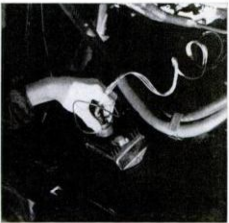
9 Plug wiring harness into control box and attach other ends as instructed.
