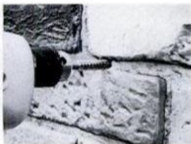
For superior holding power, drill hole in mortar joint, not brick.
