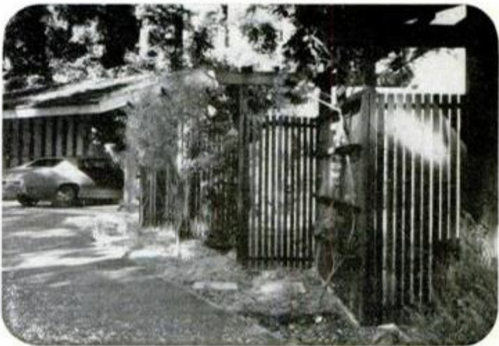
Baffle-like design breaks up strong wind currents, still lets air circulate freely.
