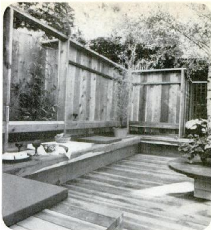
Deck wind screen with built-in benches and shrubbery niches provides solid-wall privacy for outdoor dining and leisure activities.
