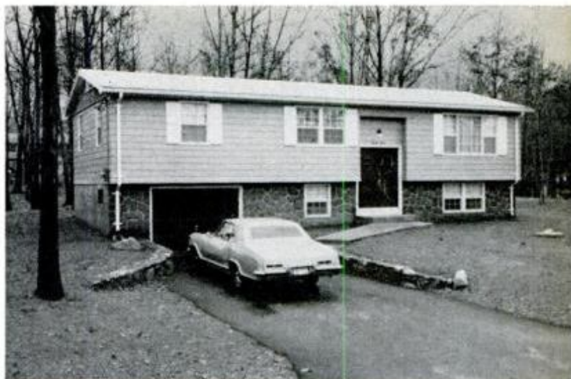
Appearances can be deceiving as here. If you hadn't seen them being built, you'd be hard-pressed to tell if these two homes were trucked in or erected on the spot. Actually, both are modulars, proving such homes can look just as normal and attractive as any conventional house.
