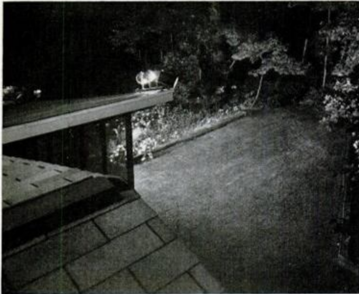
Rooftop view shows position of three 300-watt PAR units aimed at lawn and trees for dramatic effect.
