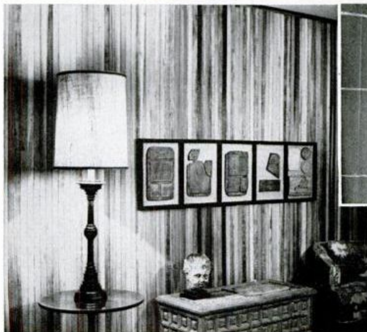
Lath in lengths of 6, 8 or 12 feet is applied to wall with panel cement or colored nails. Sand lightly, then leave it natural or coat it with satin varnish.
