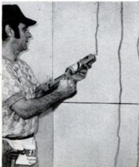
Apply adhesive liberally. Makers claim five-panels-per-cartridge coverage; professionals get two panels per cartridge.
