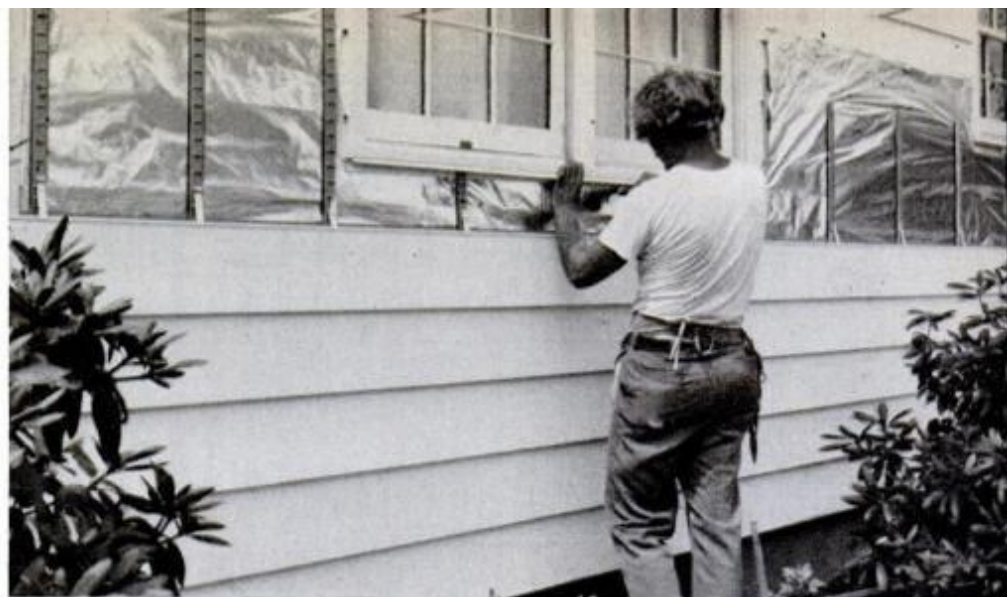
Siding system is claimed to be one-third faster than conventional way to apply siding.
