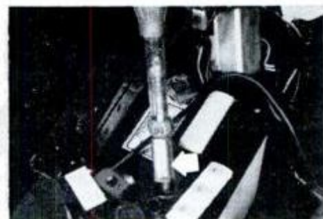
Battery electrolyte specific gravity is measure of charge and is checked with a hydrometer. This type has built-in thermometer to compensate reading according to ambient temperature.
