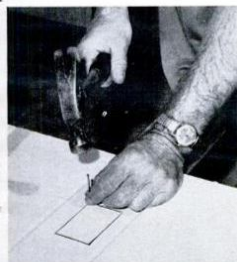
Lay panel on sawhorse table finish side up; punch holes through at four corners.
