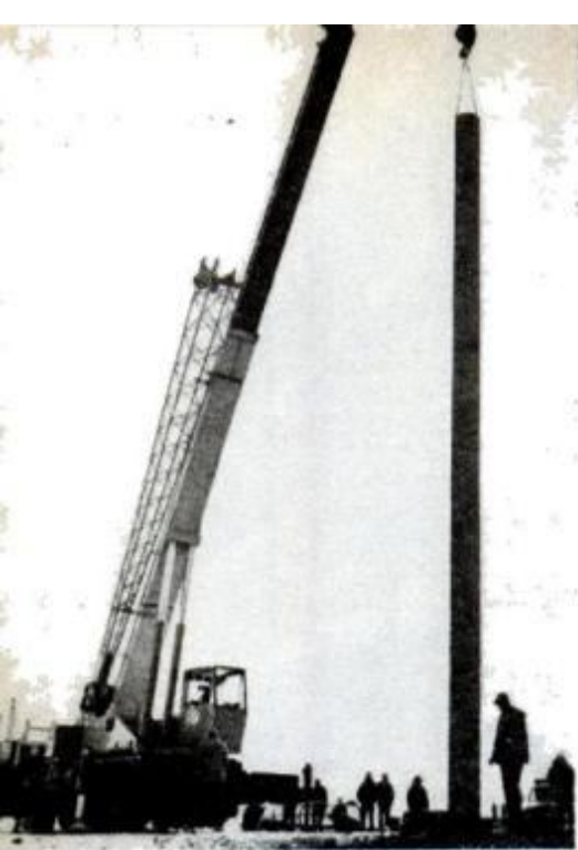
Giant mobile crane lowers 60-foot length of 18-inch pipe into ground in first stage of erecting elevated pipeline supports.
