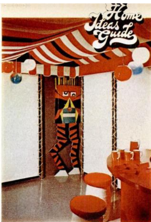
Whimsical clown-like robot in the center of the photo is simply a decorated house electric service panel. It was created by painting the conduit pipes and the box itself with bright colors and then adding a happy face. All details were carefully planned; the ceiling fixtures, for example, heighten the mood because globe shapes suggest balloons.
