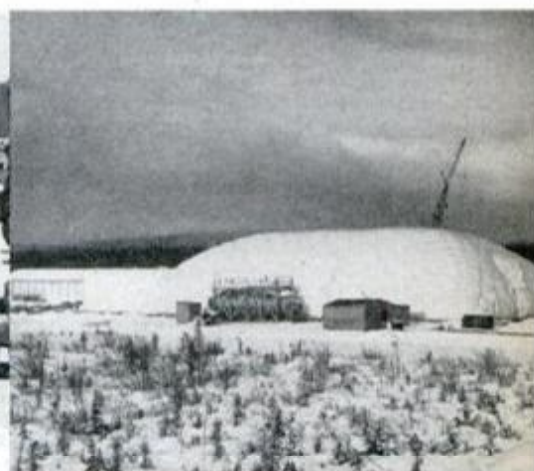
Air-inflated structure, named "Beluga" after whale it resembles, is used as temporary construction building at many sites.
