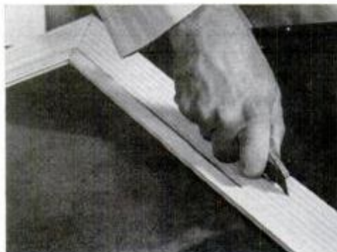
3. Use spaced \frac{1}{8} -in. grooves in plastic frame bonded to edges of safety glass as guide lines for scoring with utility knife.
