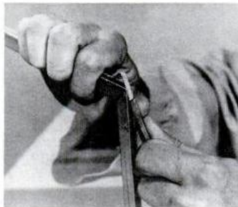
2. Remove metal frame from the old glass and save it by prying off metal clip found at each corner with a screwdriver blade.
