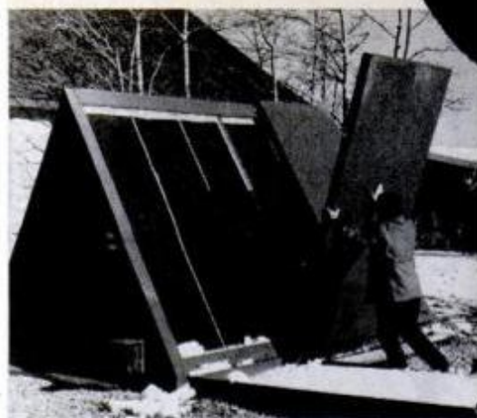
Solar "shed" can be placed anywhere in back yard, need not be built into house. Hinged reflector panels fold up (above) to protect glass-faced collectors when not in use in summer (below). Test unit here is strictly utilitarian, could be styled to look like toolshed, playhouse, mini barn, garage or other small outbuilding.
