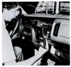
Instrument panel on Chrysler Corp. cars is accessible without dropping steering post. Handy fuse box is swing-down type.
