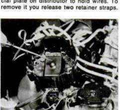
Carbon-tip center in distributor is used to make spark and ohmmeter checks since coil is packaged in the distributor cap.
