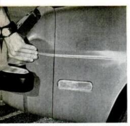
Flexible noses and tails reduce damage cost, eliminate small-nick problem. They are easily replaced by do-it-yourselfers.
