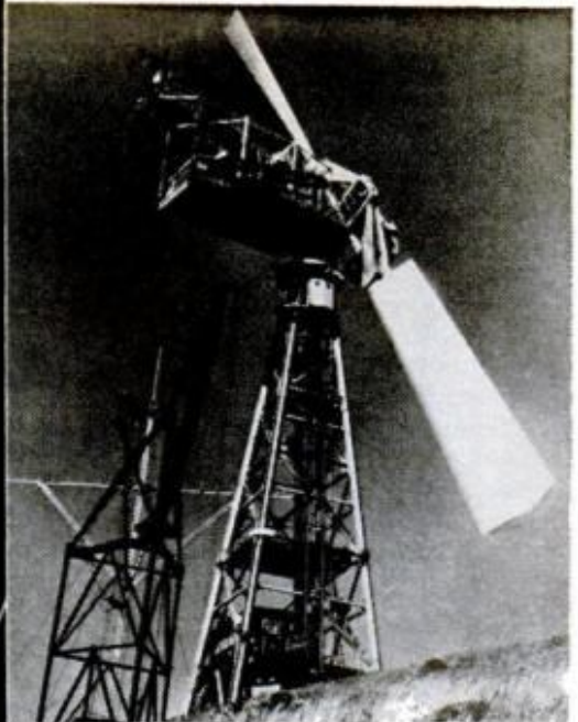
Biggest wind-power experiment to date was the 110-foot-high Smith-Putnam Wind Turbine. Located atop 2000-foot Grandpa's Knob in Vermont, the rig was in operation in the '40s. Streaks at left are star tracks caused by time exposure.
