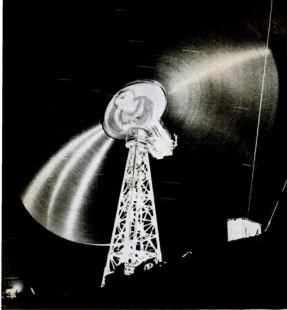
Biggest wind-power experiment to date was the 110-foot-high Smith-Putnam Wind Turbine. Located atop 2000-foot Grandpa's Knob in Vermont, the rig was in operation in the '40s. Streaks at left are star tracks caused by time exposure.
