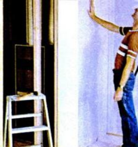
Put up gypsum wallboard.
