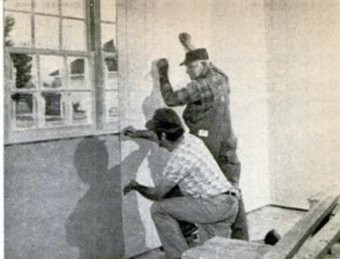
Fitting paneling around windows is done by holding panel in place and marking directly from window.
