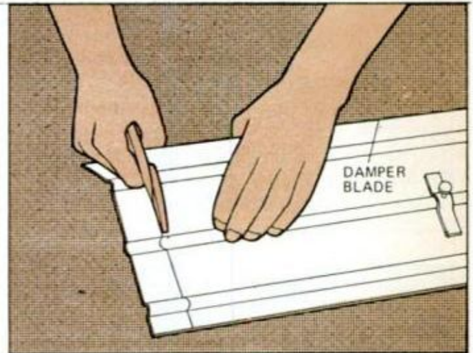
7. Trim the damper blade to duct width, allowing for a \frac{1}{8} -in. clearance at each end.
