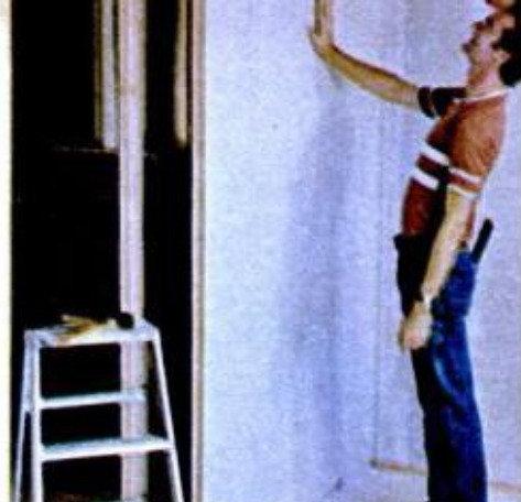
Put up gypsum wallboard.
