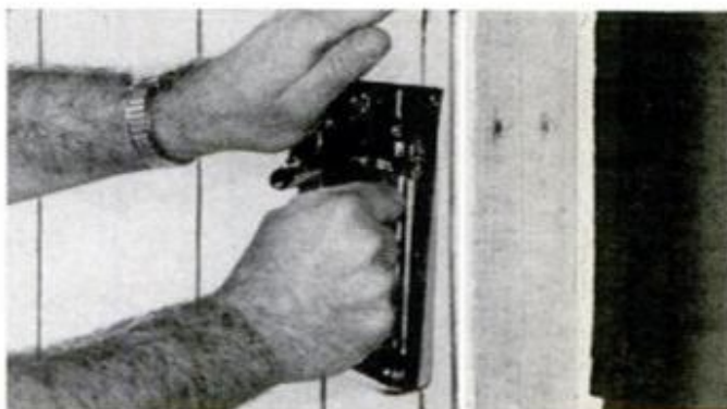
Whammer shines on paneling job. Scratches are avoided by lifting gun, instead of sliding on panel face.
