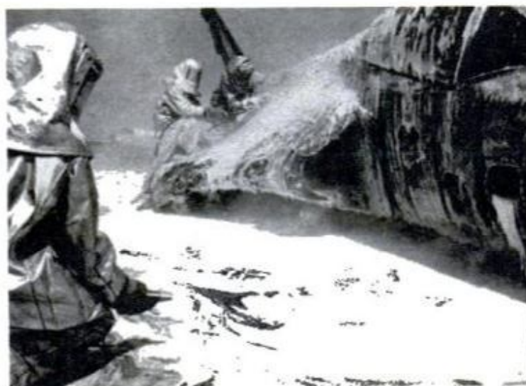
Aboard the Oriskany , men above anxiously await word of shipmates trapped in bunks by fire. Forty-four died. Below, new "lightwater" foam effectively smothers a jet fire in tests. At top right, carrier America tries out automatic flight-deck sprinkler system designed to prevent Forrestal -type disasters. At bottom right, twin nozzles can spray foam and Purple K together.
