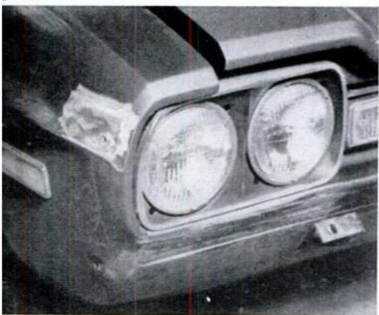
4. Always extend repair area several inches around a dent so the final filling and painting can be feathered.
