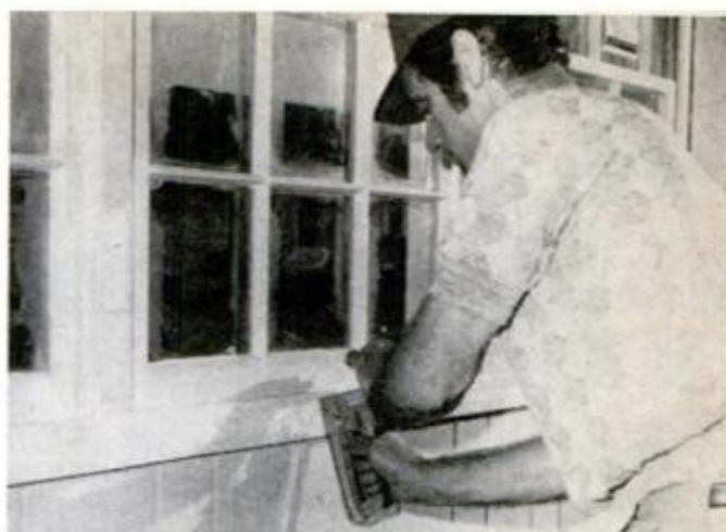
Casing can be applied using gun. Notice left-hand position to keep gun's shoe flat against the work surface.
