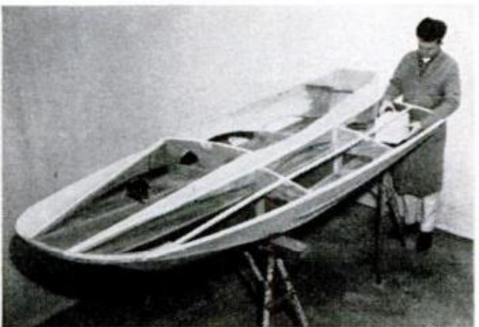
Cockpit coaming, dashboard and transom are now installed. Before decking goes on, foam flotation material can be fitted into void areas for strength, safety.
