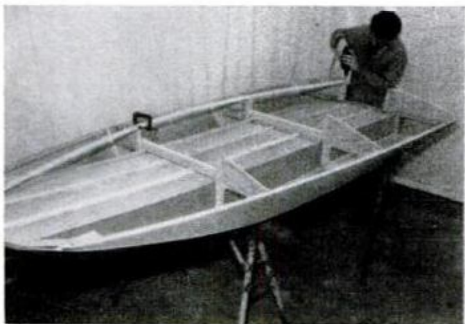
Deck framing members are installed after hull is planked and righted. Carling is positioned in notches in frames, transom. Note notches, blocking for battens.
