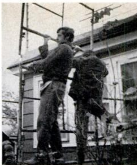
Scaffolding required a bit of jiggering on this side of house because of cantilevered window section in rear. It took three men 20 minutes to assemble.
