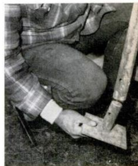
Because ground is level , rigid base-plates were used. If grade is uneven, leveling-type jack-plates must be used to keep scaffolding level, plumb.
