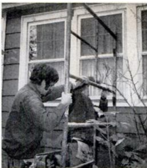
Scaffolding required a bit of jiggering on this side of house because of cantilevered window section in rear. It took three men 20 minutes to assemble.
