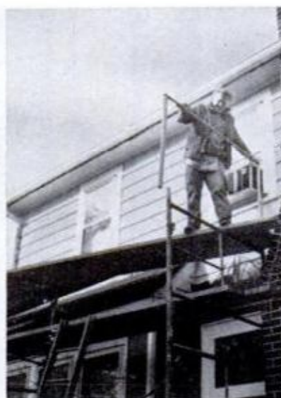
Ladder is used to reach peak at gable end. It, in turn, rests upon plank held by roof brackets fastened to porch roof.
