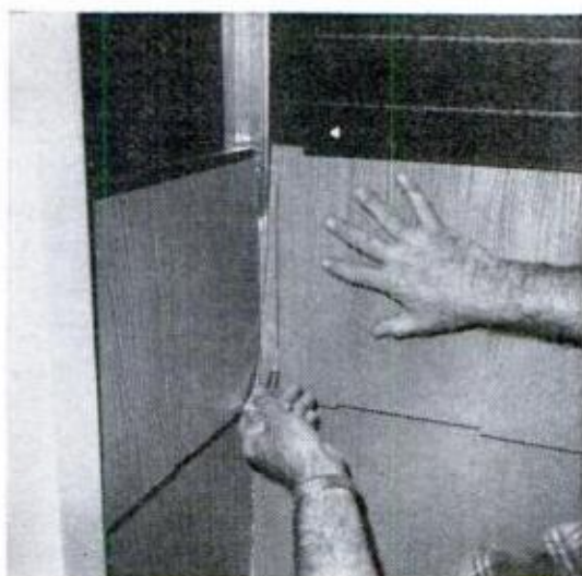
Second shingle is held in place and scribed for custom fit. To see finished inside corner, see photos at top of page 99.
