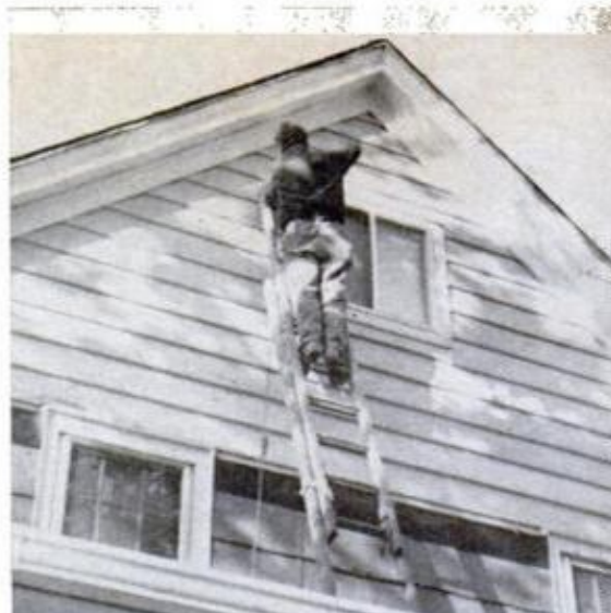
Ladder is used to reach peak at gable end. It, in turn, rests upon plank held by roof brackets fastened to porch roof.
