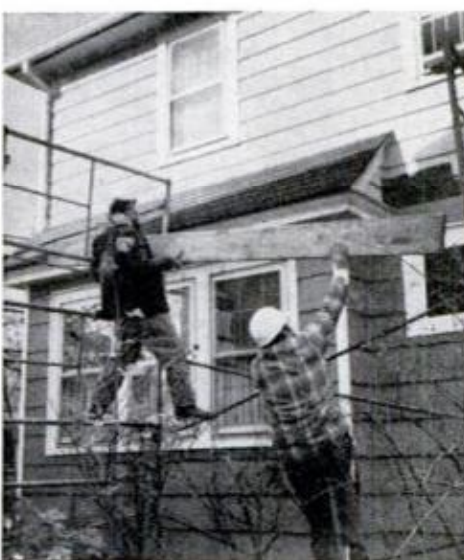
Two pairs of diagonal braces are used between each pair of platform end frames. Until diagonal braces are secured, the insert-pins keep sections from falling.
