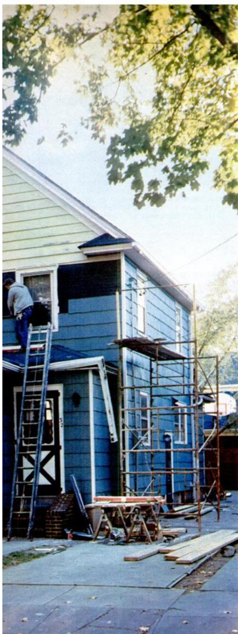
Before and after photos taken during the first and last weeks of November. Original clapboard siding was cracked, blistered and peeling (turn page for close-up look). New siding enhanced looks, reduced fuel consumption.
