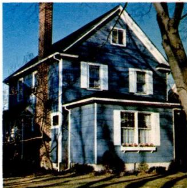
Before and after photos taken during the first and last weeks of November. Original clapboard siding was cracked, blistered and peeling (turn page for close-up look). New siding enhanced looks, reduced fuel consumption.
