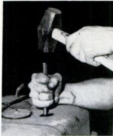
Punch a 3/8-inch hole in the tank so that chassis punch can be used.
