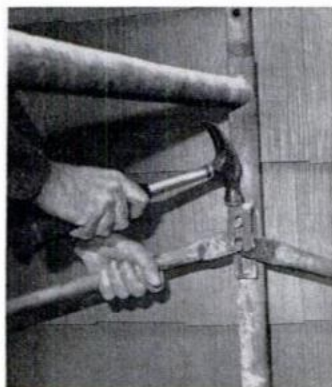
Diagonal brace is slipped over stud on platform leg (left) and the brace-lock is tapped into lock position. Center: Brace stays put until you remove it.
