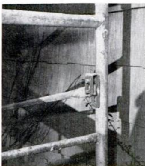
Diagonal brace is slipped over stud on platform leg (left) and the brace-lock is tapped into lock position. Center: Brace stays put until you remove it.
