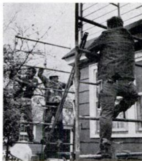
Two pairs of diagonal braces are used between each pair of platform end frames. Until diagonal braces are secured, the insert-pins keep sections from falling.
