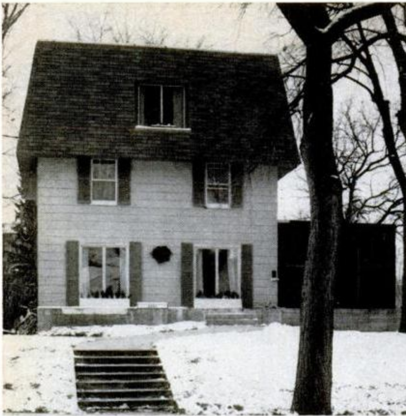
Front of house (above) with third story and new mansard roof added. Family room, under construction at right, will have mansard roof to match. Rear view (below) shows recessed balcony in third story, new dining-room addition, sun deck and family room being added.
