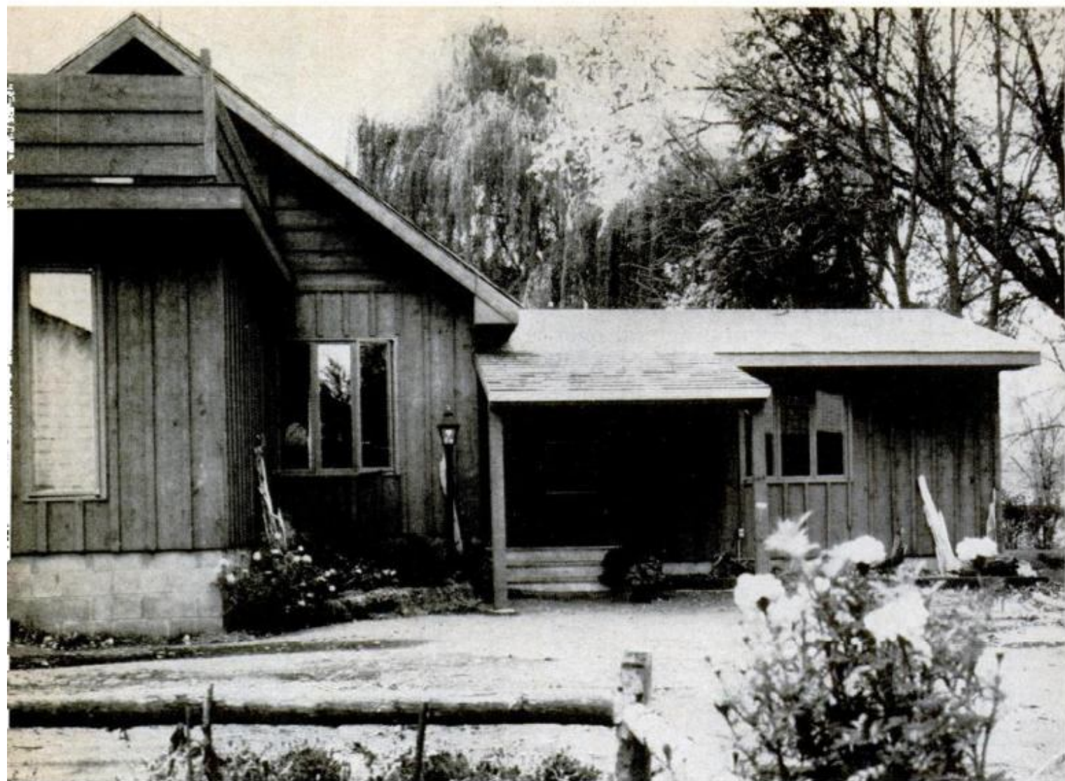
Handsome new exterior features rough-sawn cedar board-and-batten siding that replaced white clapboard of old.
