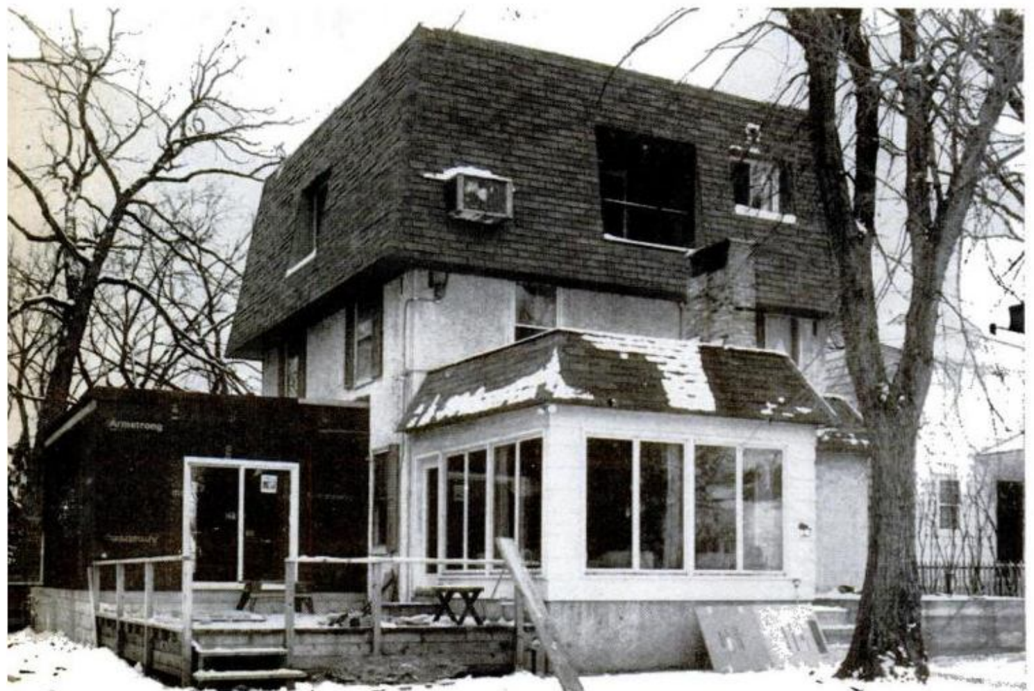
Front of house (above) with third story and new mansard roof added. Family room, under construction at right, will have mansard roof to match. Rear view (below) shows recessed balcony in third story, new dining-room addition, sun deck and family room being added.
