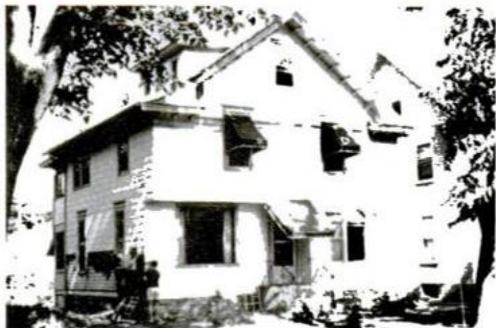
Exterior of 75-year-old home was rejuvenated by replacing old white asbestos shingles with stained cedar shakes.
