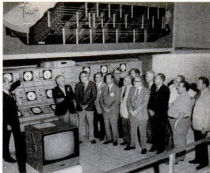
Training in loading and cargo handling is provided by long control panel and display board showing a hypothetical tanker configuration. Computer-controlled, board shows if pumps are working, if valves are open or closed, type and level of cargo in 23 tanks.
