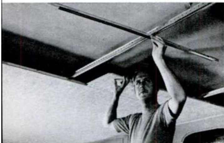
Suspended ceilings with hidden support
