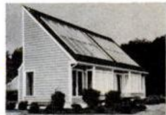
Switching on the sun . . . 190
