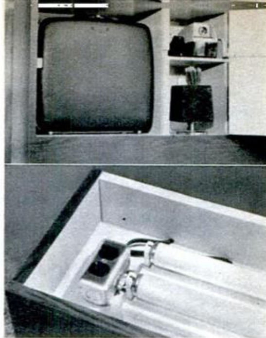
Wall cabinet stores typewriter, other supplies (top photo). Lower photo shows recess in underside of cabinet for a fluorescent light controlled by main switch in outlet box.
