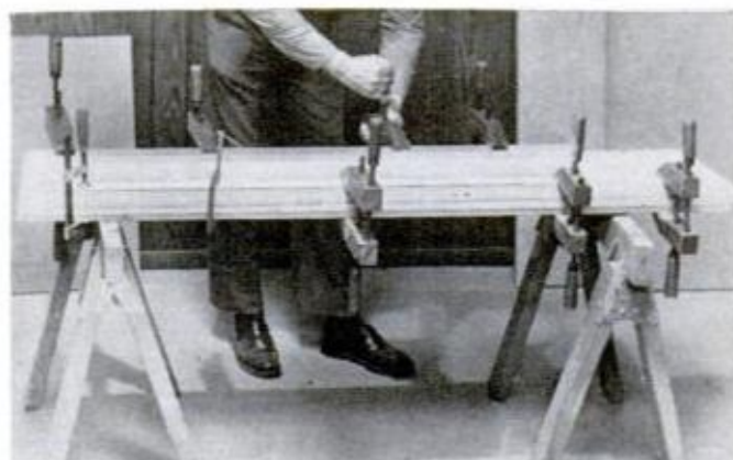
Doubled-up plywood panels achieve thickness of 1½ in. To assemble the panels, use screws and glue.
