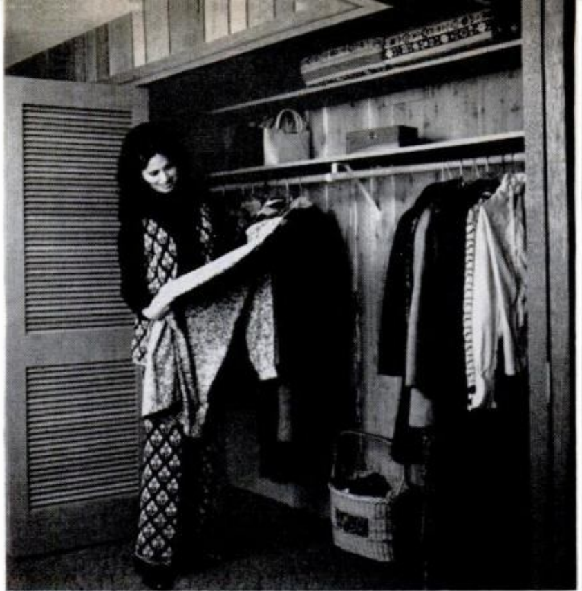
Plywood liner makes instant cedar closets
