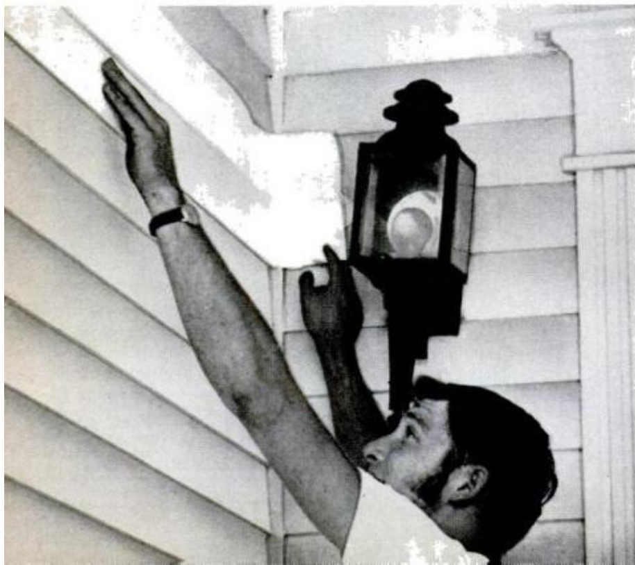
Vinyl siding is 'house paint' you press in place
