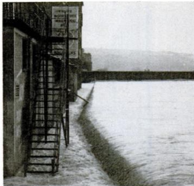
Elmira's north-side flood wall was a huge spillway at 9:00 a.m., June 23. The rush of water was part of the worst flood in the state's history.
