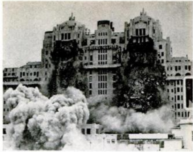
TWO CENTER WINGS are first to go (right), leaving Traymore's twin-domed main section ready for removal in second stage (shown on preceding pages). Debris was cleared away after each stage to make room for more to come in the following stages, simplifying the cleanup job. (Photos above and below by Ken Sooy)
