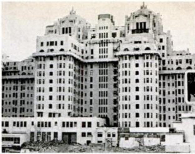
TWO CENTER WINGS are first to go (right), leaving Traymore's twin-domed main section ready for removal in second stage (shown on preceding pages). Debris was cleared away after each stage to make room for more to come in the following stages, simplifying the cleanup job. (Photos above and below by Ken Sooy)
