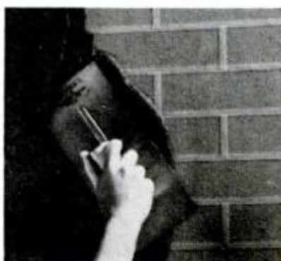
8 TROWEL FINISH COAT (Formula II) over wall and tape; allow mixture to dry 2 to 4 hours
