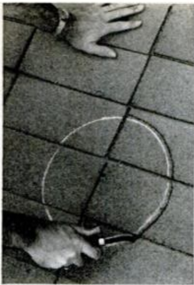
3. USING CIRCLE AS A GUIDE, cut away shingles with sharp knife. Cut \frac{1}{2} in. outside circle
