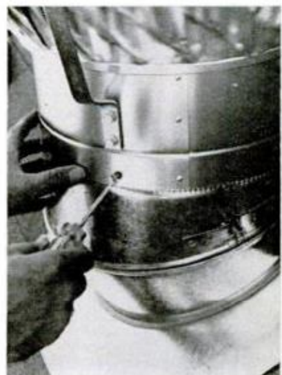
11. LOCK RING TO FLANGE with No. 8, \frac{1}{2} -in. sheet-metal screws. Drive screws home for tight fit
