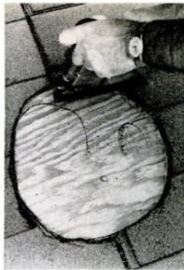
4. CUT HOLE through roof boards with sabre saw or by hand with keyhole saw, following the circle
