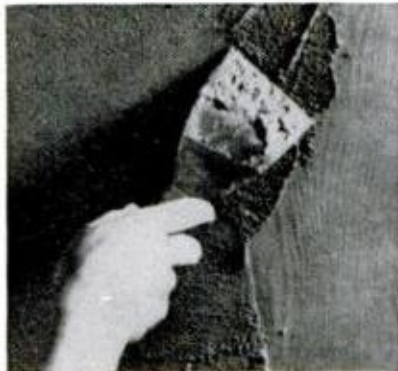
1 USE TROWEL or wide putty knife to apply thin layer of base coat (Formula I) on wall
