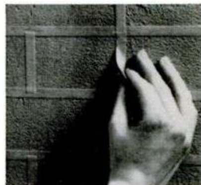
6 WITH RAZOR BLADE, cut vertical tapes at center where they cross each horizontal tape strip
