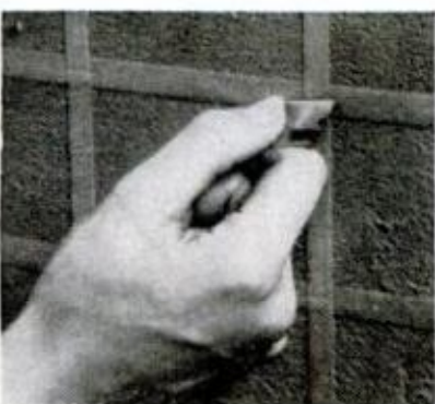
7 FORM BRICK SHAPES by removing every other vertical tape in each row or brick course
