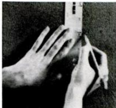
2 LET DRY OVERNIGHT; use trowel to scrape off roughness, ruler to mark wall vertically
