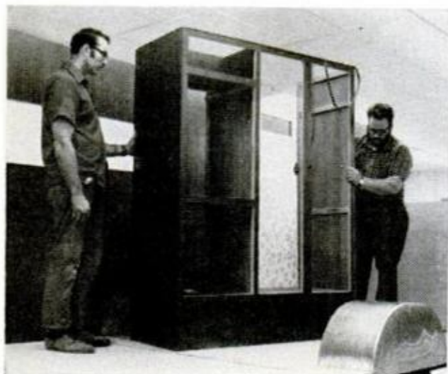
WALLS are framed out with 2x2s, paneling is glued and stapled or nailed. Panel bit routs edges, windows
