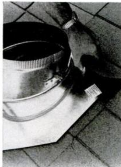
7. RETIGHTEN SCREW, then slide top half of flashing up under shingles, removing nails in way
