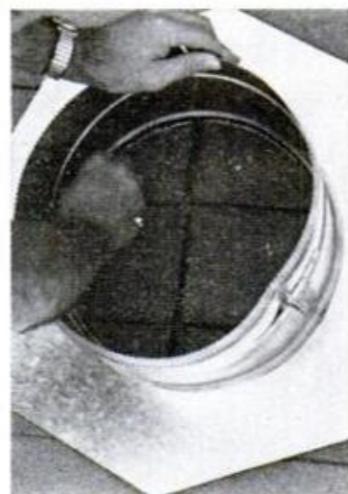
2. CENTER BASE over pilot hole in roof and use inside of base to scribe hole on roof shingles
