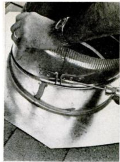
5. WITH SCREWDRIVER, loosen the locking screw on adjustable-pitch base so you can turn it
