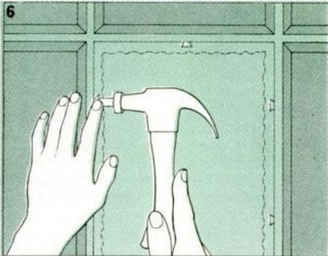
6 Drive glazier's points, size 1 or 2, using driving tool packaged with points. On small pane use one point along short sides of glass, two on long.
