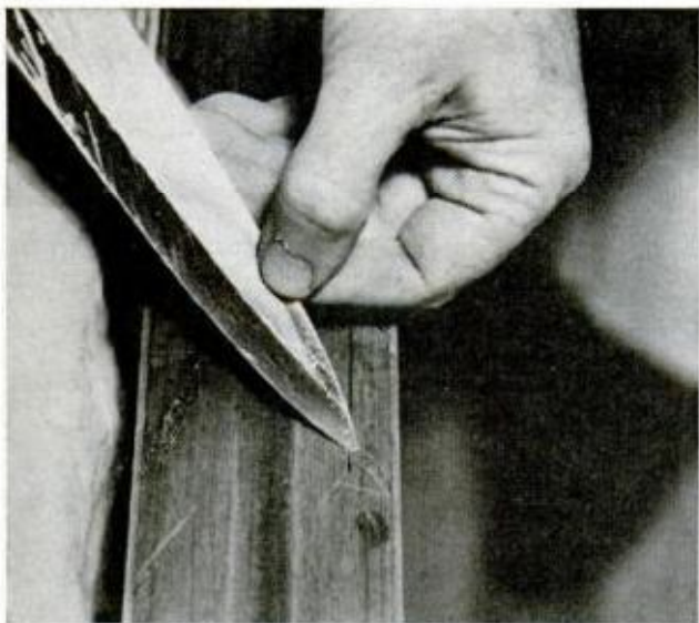
DEEP GOUGES require more than waxing to fill and repair. First use knife or other sharp tool to dig out any loose foreign matter before starting repair
