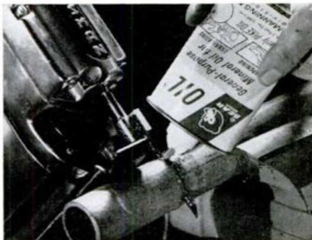
WHEN POWER-HACKING PIPE or angle iron, use the saw's slowest speed and flood the cut with light oil
