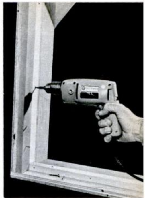
SCREWDRIVER BIT in a variable-speed drill makes quick work of driving home the many screws needed
