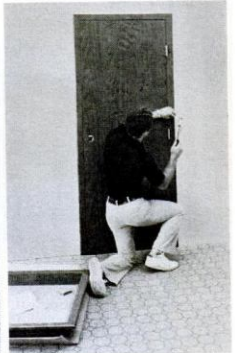
Nail and shim the door and jamb into the wall opening.
