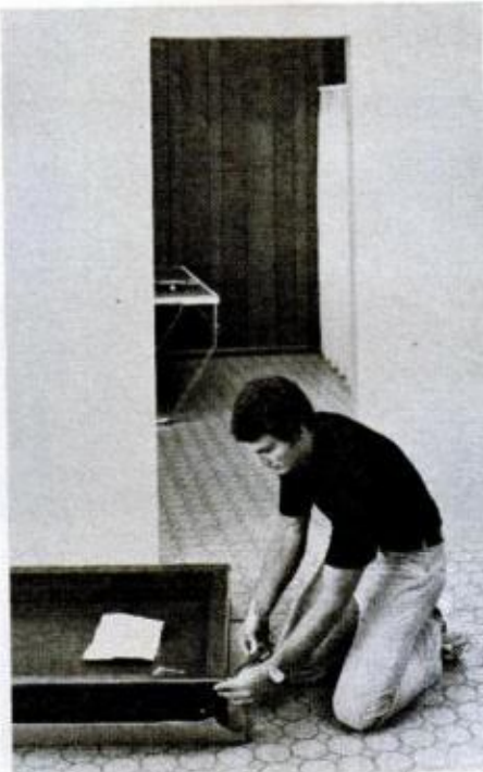
Screw the top of the casing to the sides.
