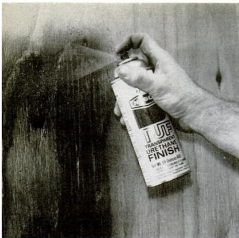
UNIQUE TRANSPARENT FINISH is easy to apply, it can be used on glass and metals as well as on wood
