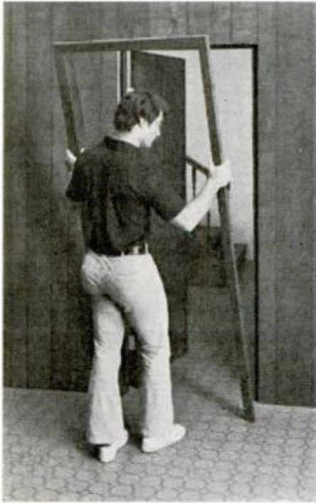
On the other side, slide assembled casing into jamb and nail.
