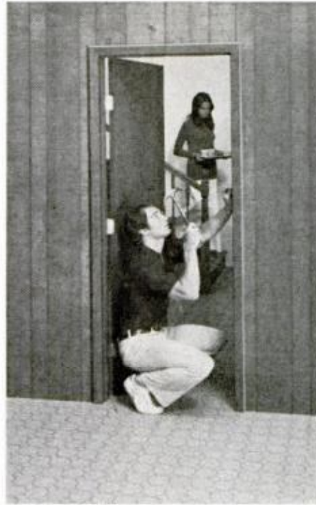
Nail through stop, jamb, and casing extensions to lock entire unit together and into wall.
