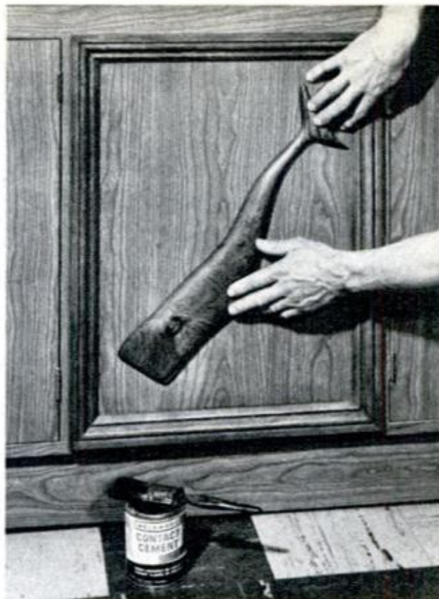
BAS-RELIEF CARVING is cemented to center frame as decorative touch. Contact cement secures it to slick laminate, or it can be screwed on from back
