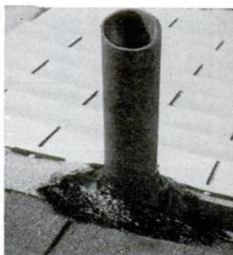
PLASTIC ROOF CEMENT is used to seal the joint around stack in roof. Cement is applied with a putty knife (a wood shingle will work fine) after shingles are trimmed for a neat job. If desired, paint cement
