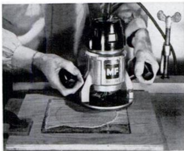
ROUTER CUTS RECESS in cabinet top to hold metal plate against which the router base will be clamped
