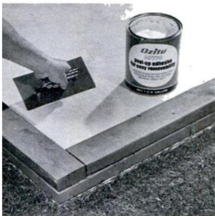
USE NOTCHED TROWEL to spread adhesive on area of exposed widths. When almost dry, turf goes down AUGUST 1972
