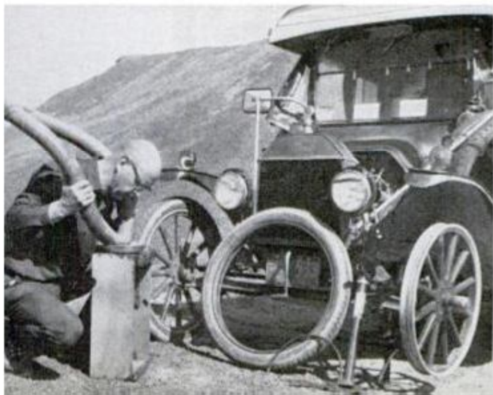
LAST OF TRIP'S THREE FLATS was discovered on the morning of final day out. Locating a slow leak in tube called for an improvised water immersion test
