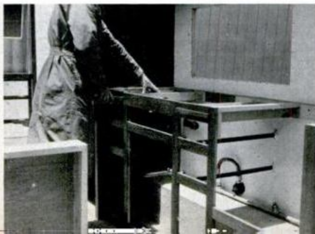
KITCHEN SINK CABINET is shop-assembled, positioned in trailer after rough-in plumbing is installed
