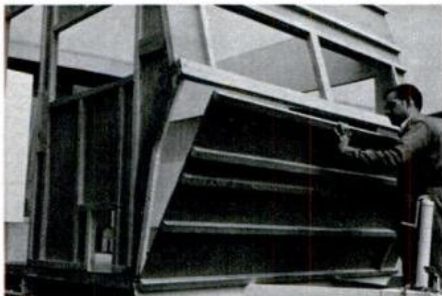
WHERE TOP AND BOTTOM parts of front wall butt, V-cavity is filled with wedge-shape piece of wood
