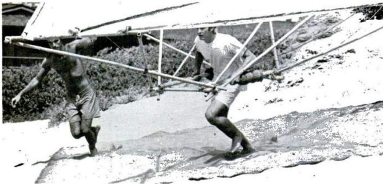
POISED FOR TAKEOFF , kiteman above begins run down slope that will lift him into air. Below are two harness arrangements. At left, pilot hangs vertically in parachute-like straps; at right, rider sits in a sling
