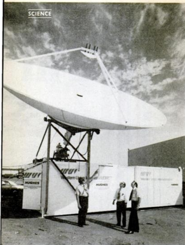
GROUND STATION was flown to Peking prior to the President's visit. Made by Hughes Aircraft, the facility boasts a 24-foot-diameter antenna and enough electronics to transmit 1 color TV broadcast, 9 voice commentaries and 60 two-way phone conversations. It beamed transmissions to Intelsat IV, as shown in the drawing
