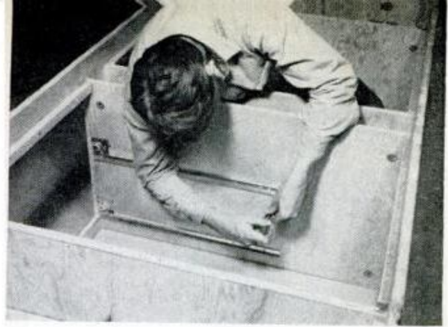
DRAWERS ROLL SMOOTHLY on standard metal guides which are screwed to the dividers and drawer sides
